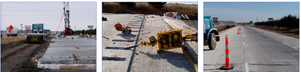
Figure 7. Installation of the precast panels at the Missouri project (left, staging of trucks and installation crane; center, final post-tensioning; right, completed project).
