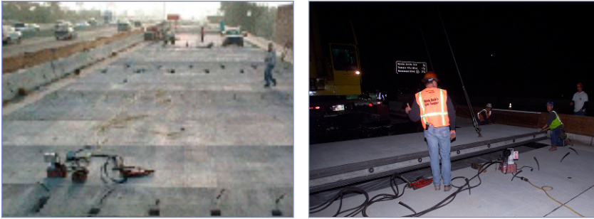
Figure 6. PPCP installation along I-10 in El Monte, California.
