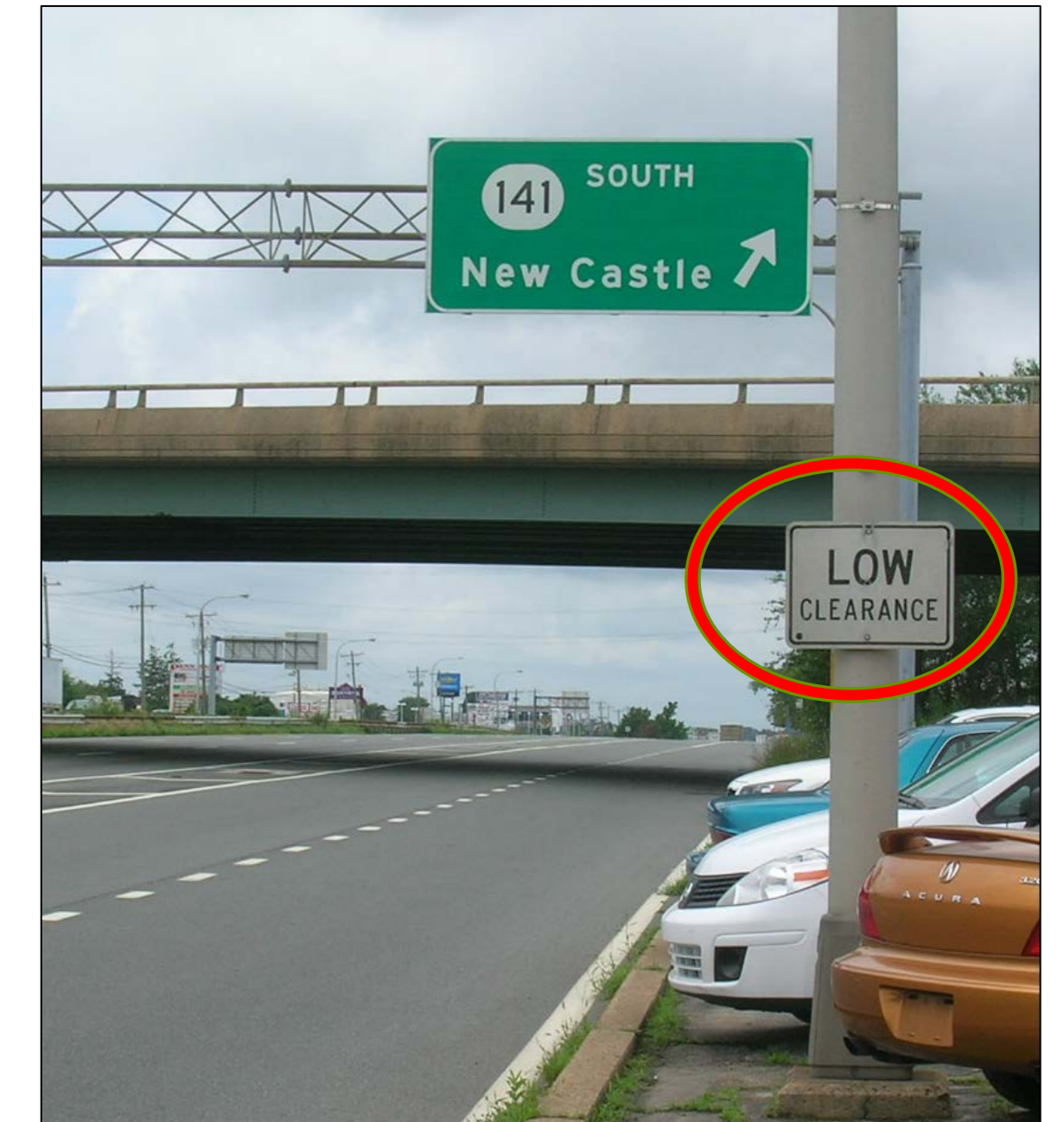
Looking SB on US 13
