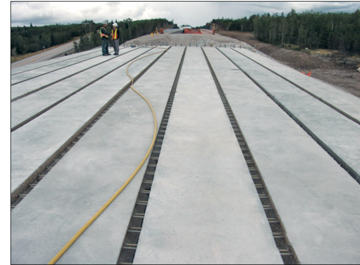
UHPC – Hawk Lake Bridge (Ontario, Canada) Ref: Precast.org
