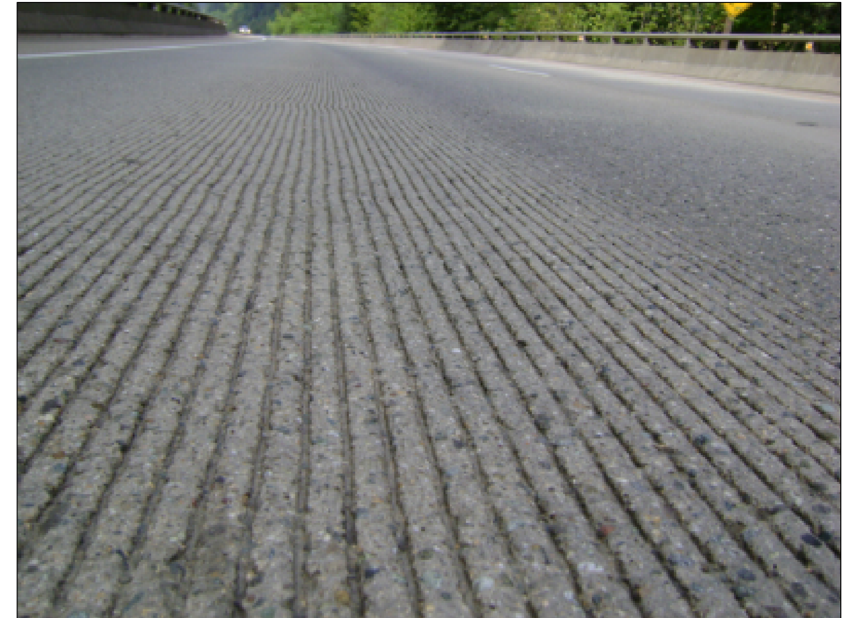
Oregon DOT Eagle Creek Viaduct – PPC Overlay Ref: Kwik Bond Polymers
