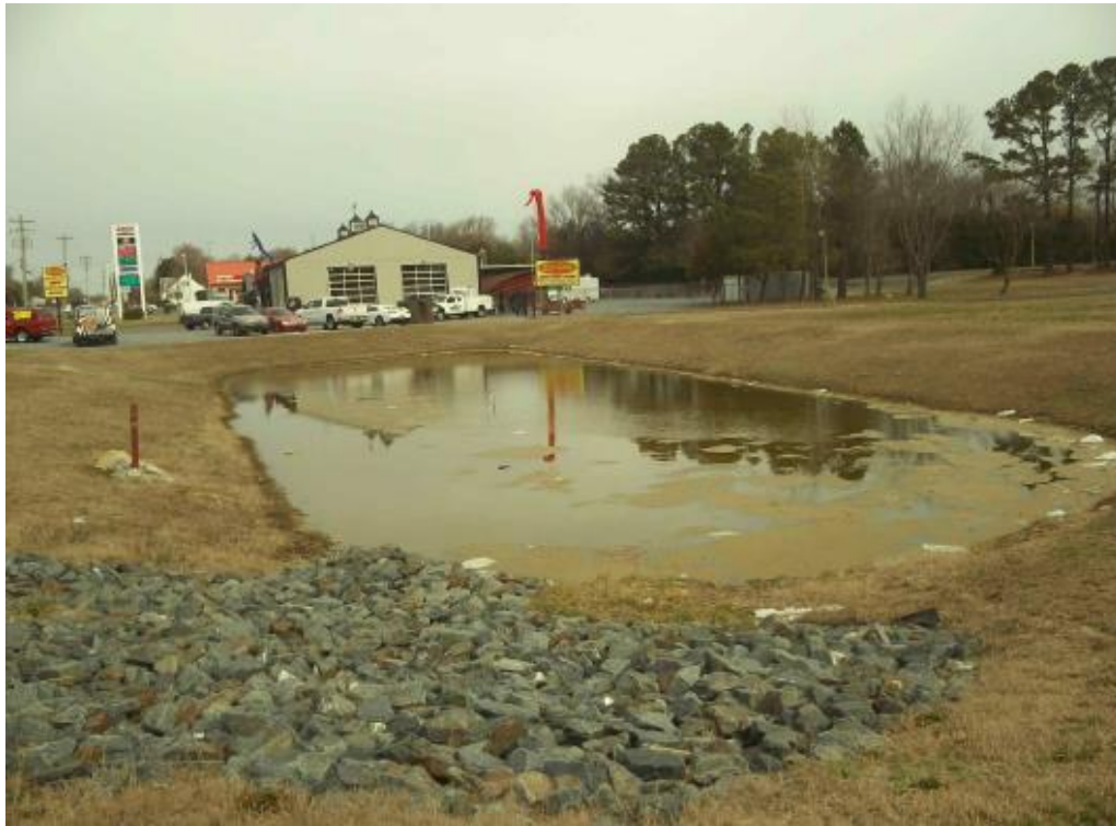
BMP 883 – SR 1/Thompsonville
