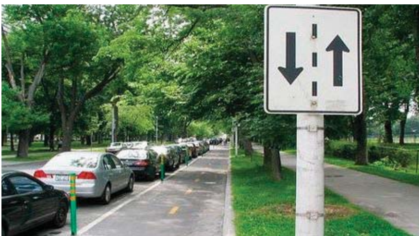
Figure 3.4-5 Separation for All Users with Parking
