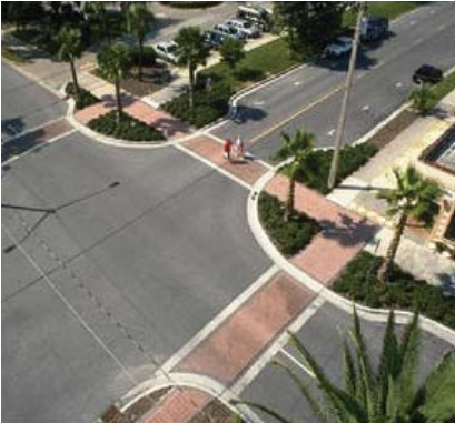
Figure 3.11-2 Curb Extensions/ Neckdowns
