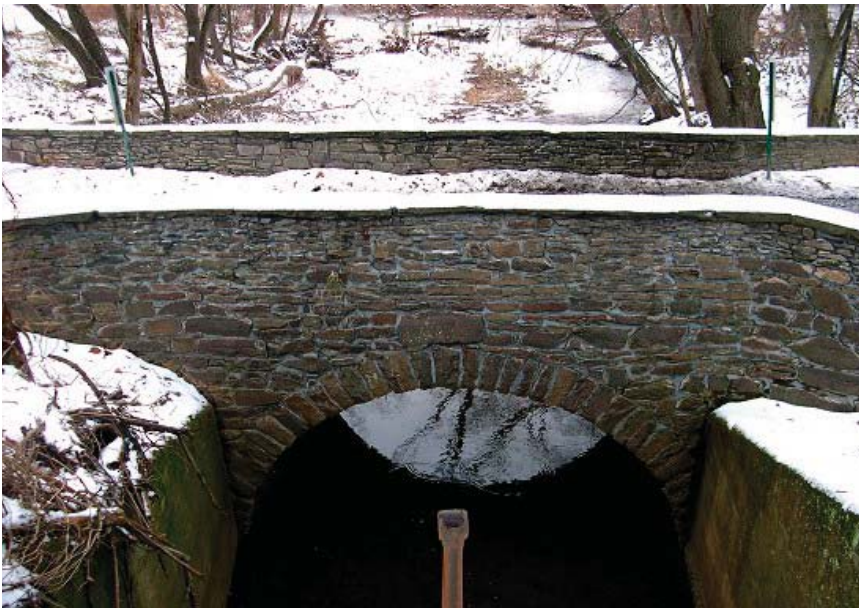
Figure 3.3-1 Bridge: Stone at D&R Canal State Park, NJ
