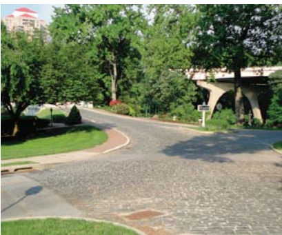
Figure 3.11-4 Use of Paving Stones or Cobblestones
