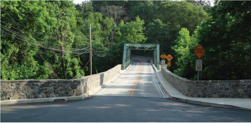
Figure 3.2-3 Guardwall: Stone-Faced, Bridge 1 over Brandywine Creek, Wilmington, DE
