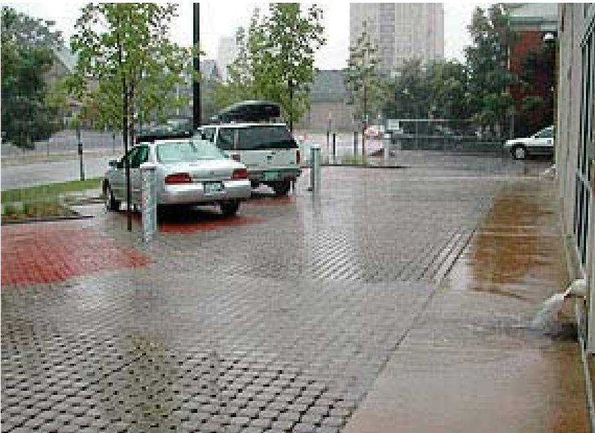
Figure 3.5-6 Sidewalk Permeable Treatments
