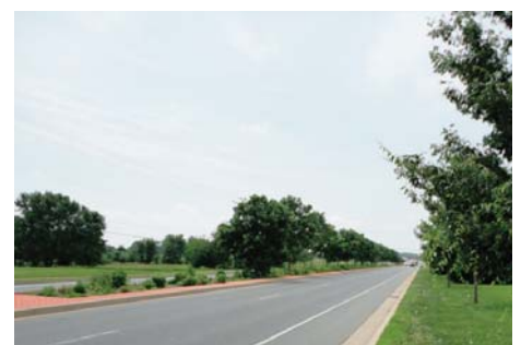
Figure 3-1 Design Flexibility: Narrow Lanes to Provide Median, SR 7 Bear, DE
