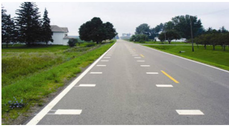
Figure 28 Transverse markings used to induce slower operating speeds (Source: FHWA)
