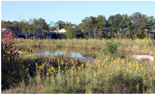
Figure 51 Example of a stormwater management facility designed to reinforced the natural character of local wetlands through the use of native wetland plant species
