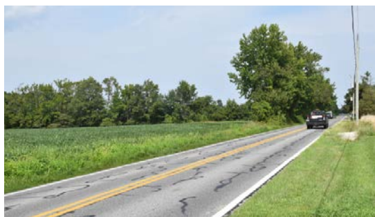
Figure 2 New Road near Lynne Road intersection
