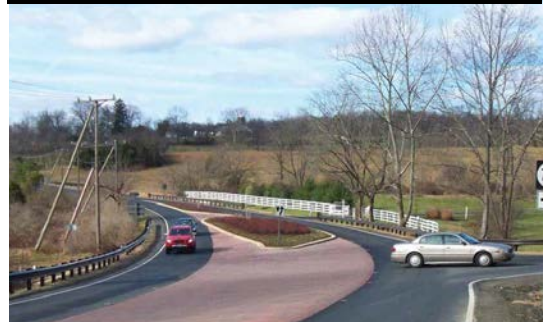
Figure 72 Splitter with pavers at intersection
