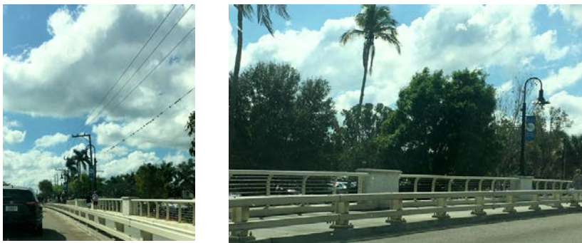
Figure 85 Box beam (inside) and pedestrian railing exemplify the preferred railing type
