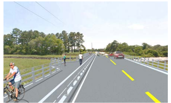
Figure 87 Illustrative concept showing a combined structure used to accommodate both the vehicular travel lanes and the shared use pathway with an overlook to Canary Creek
