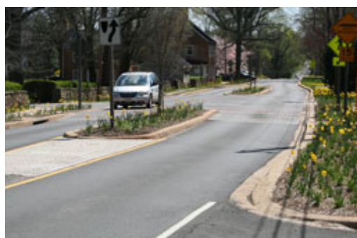
Figure 80 Narrow splitter island with crossover
