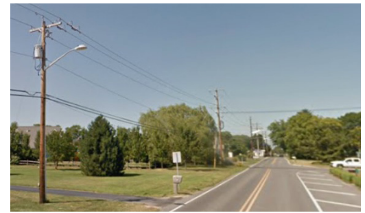
Figure 58 Existing roadway lighting on New Road is limited to the section between 4th Street and Pilottown Road (including approach to 4th Street shown above)
