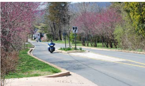
Figure 30 A splitter island combined with landscape roadside plantings effectively reduce operating speeds on U.S. Route 50 in Virginia (see Figure 33)
