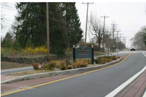
Figure 31 Combined splitter island and gateway approaching Centreville, DE on the Brandywine Valley National Scenic Byway and Harriet Tubman Underground Railroad slows traffic while increasing visual appeal, as noted in the visual preference survey
