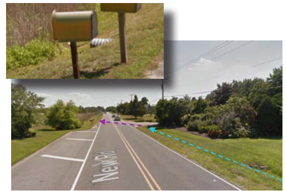
Figure 92 Ditchline on WB side of New Road leading to outlet on EB side (inset)
