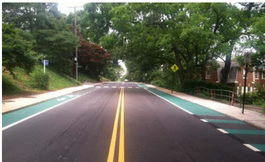
Figure 63 Where bicycle lanes are added on New Road to meet the requirements of Delaware's Complete Street Policy, green painted lane markings should be considered to differentiate between the travel lane and bicycle lane especially approaching the more urban sections with many intersections and driveways
