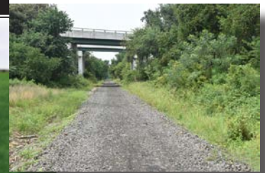
Figure 68 DeIDOT concept utilizes the existing bridge parapet and bridge columns without modification. The rail-trail, relocated to the outside of the existing columns, will require a low retaining wall
