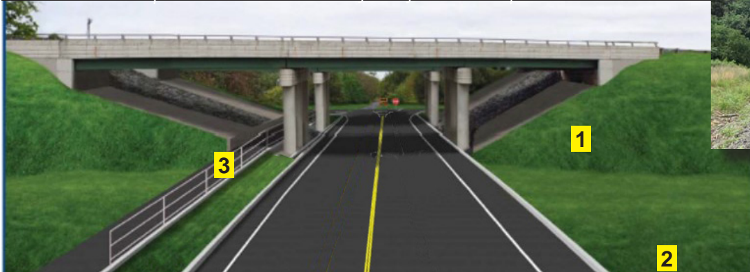
Figure 68 DeIDOT concept utilizes the existing bridge parapet and bridge columns without modification. The rail-trail, relocated to the outside of the existing columns, will require a low retaining wall
