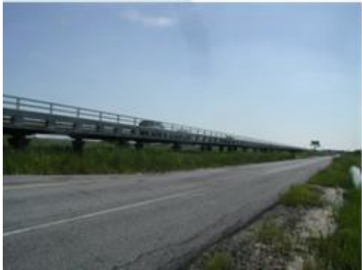
RAISED & REROUTED ROADWAYS STATE ROUTE 54, SUSSEX COUNTY, DELAWARE
