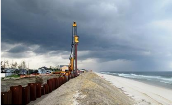
BURIED FLOODWALL / STRUCTURAL DUNE MANTALOKING, NJ, MOTT MACDONALD
