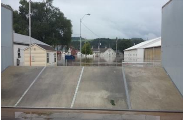
PERMANENT DEPLOYABLES FLIP UP GATES BLOOMSBURG, PENNSYLVANIA
