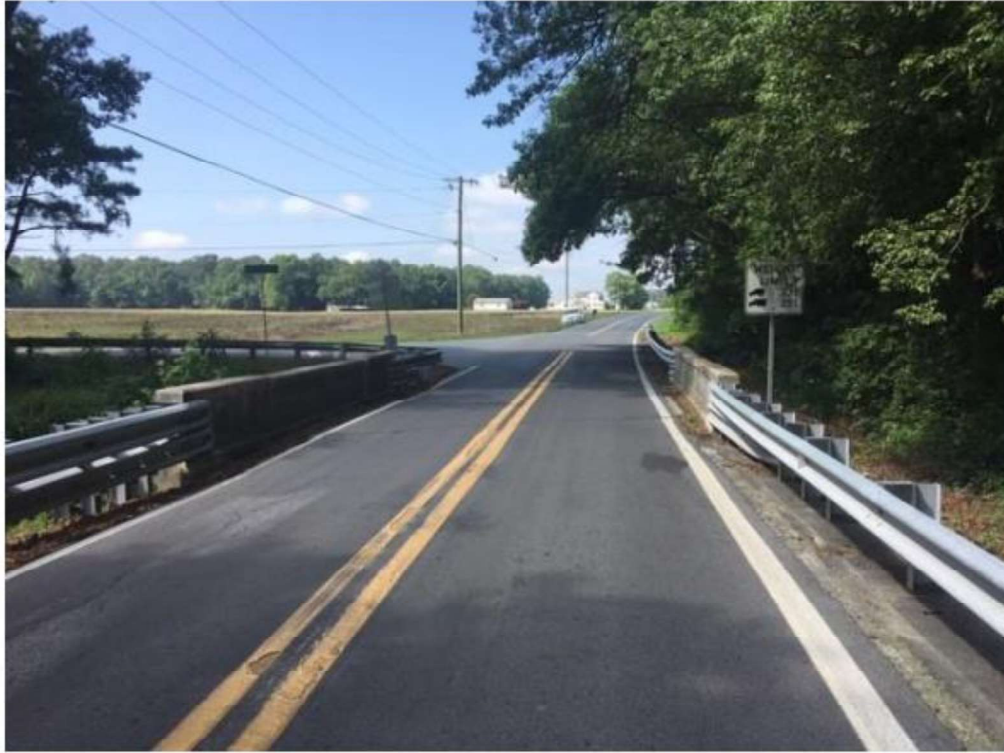
Photo 3 NORTH BRIDGE APPROACH POSTING SIGN
