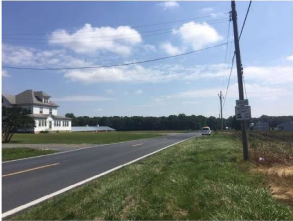
Photo 1 POSTING SIGN ALONG WOODPECKER RD WEST OF BUTLER MILL ROAD
