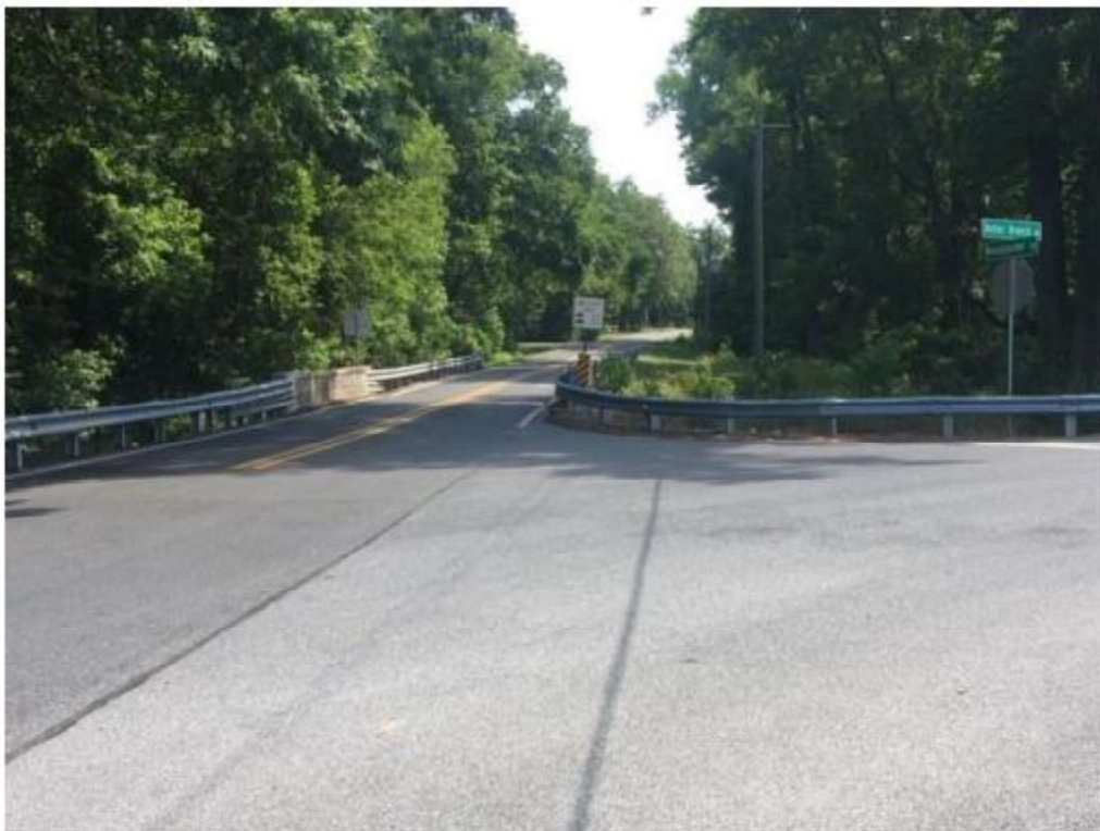
Photo 2 SOUTH BRIDGE APPROACH POSTING SIGN
