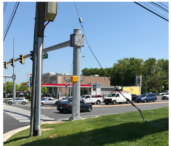
Figure 9-2: Guy anchor and wire supporting utility pole.
