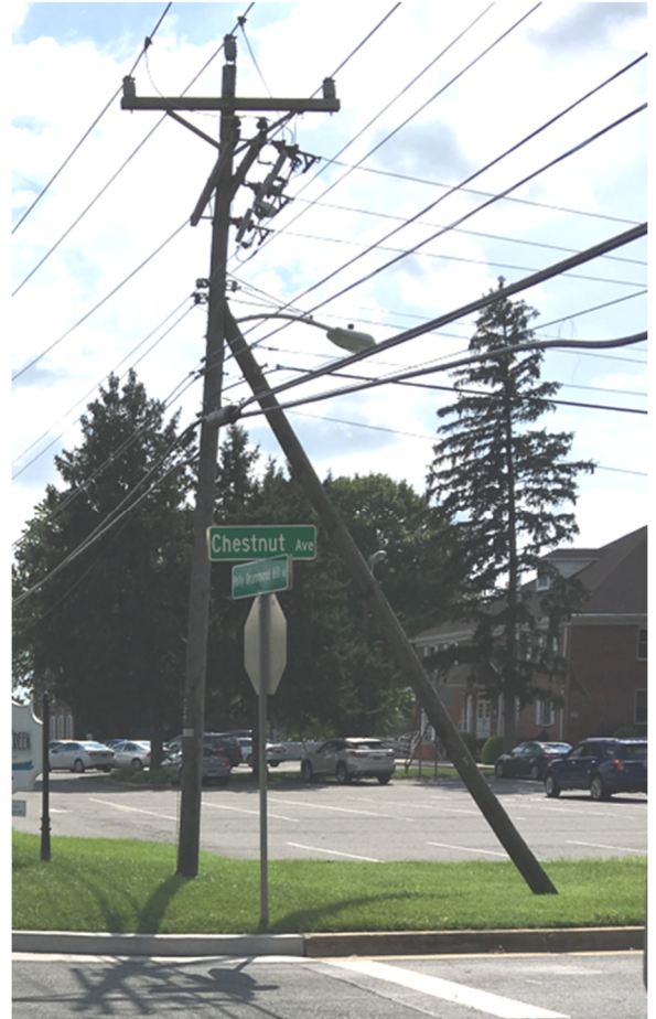
Figure 9-1: Push pole bracing Delmarva Power utility pole.
