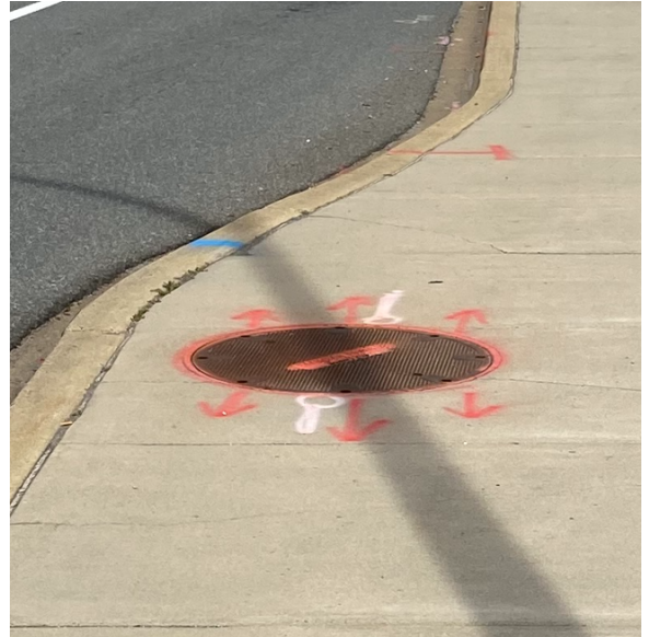
Figure 10-1: Delmarva Power manhole lid in sidewalk with Miss Utility markings for adjacent underground facilities.
