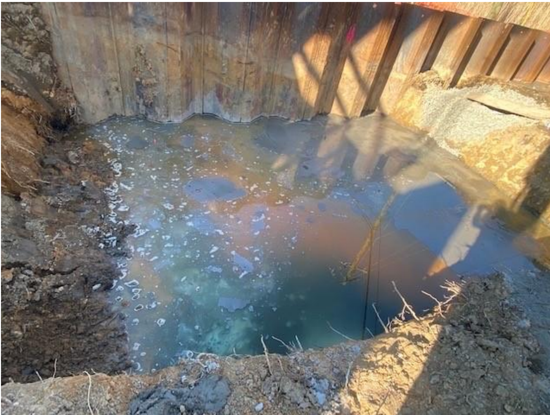
BR 159, James Street Bridge Project
