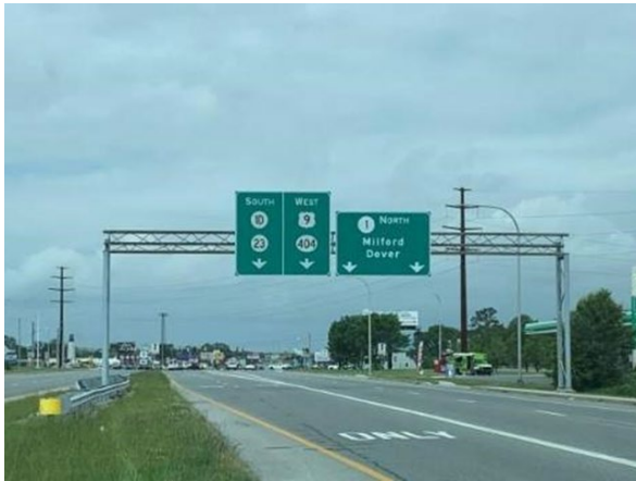
Northbound SR 1 left turn lane signing
