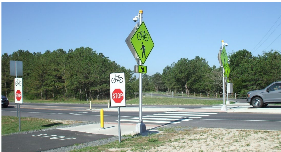
Rectangular Rapid Flashing Beacons (RRFBs) on Freeman Highway
