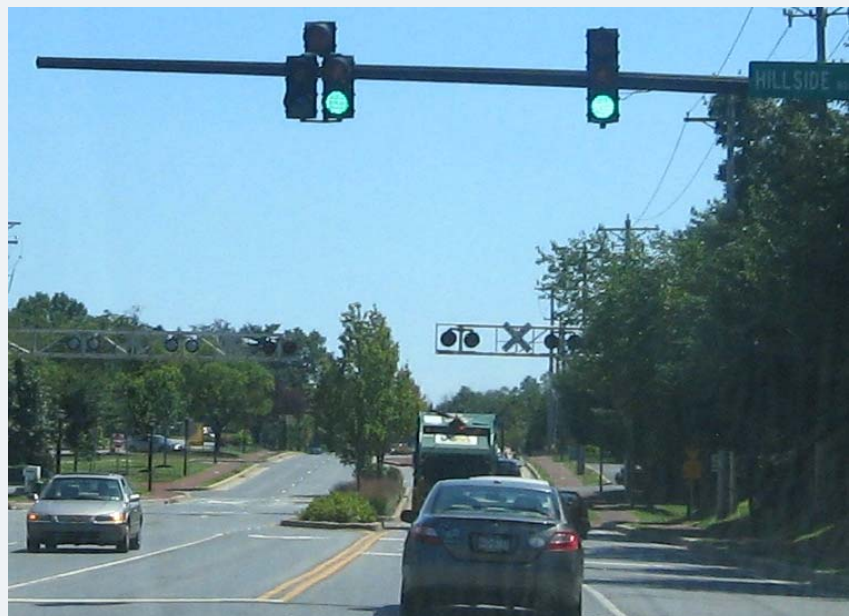
SR 52 at Hillside
