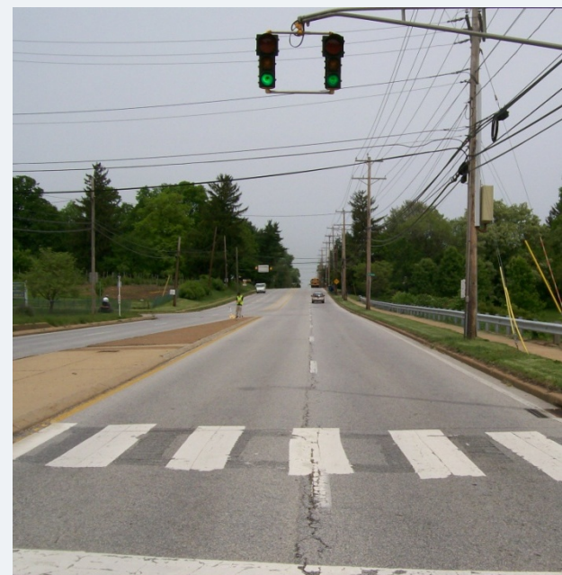
Faulk Rd Mid-Block Crossing @ Brandywine H.S.
