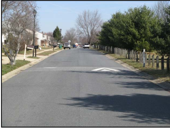
SPEED HUMP (Valley Forge Road)
