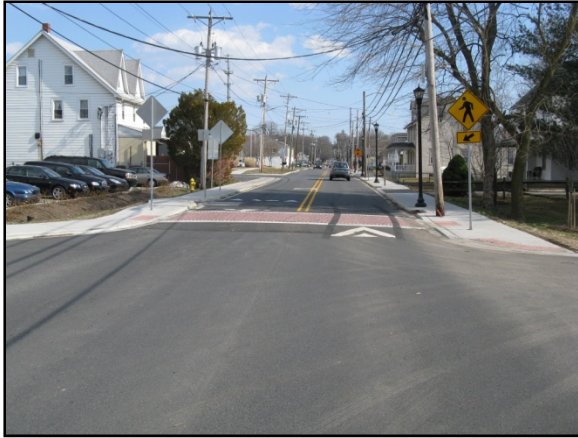
RAISED CROSSWALK (Old Lancaster Pike)
