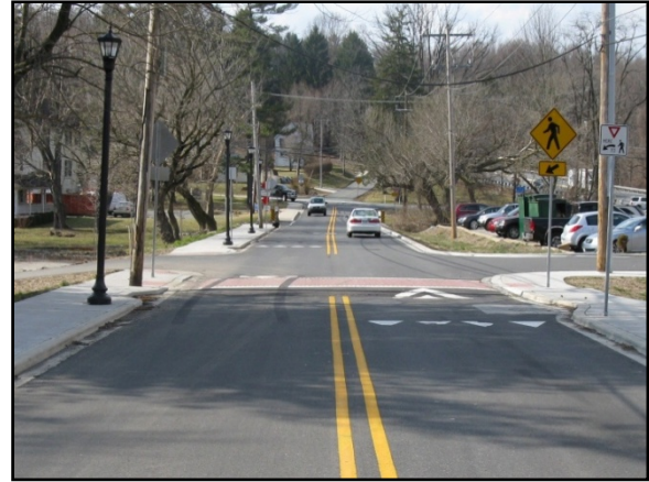
RAISED CROSSWALK (Old Lancaster Pike)
