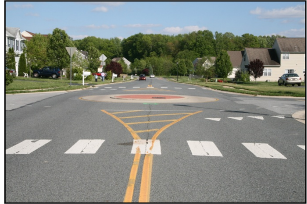
MINI-ROUNDABOUT (Rose Hill Drive)
