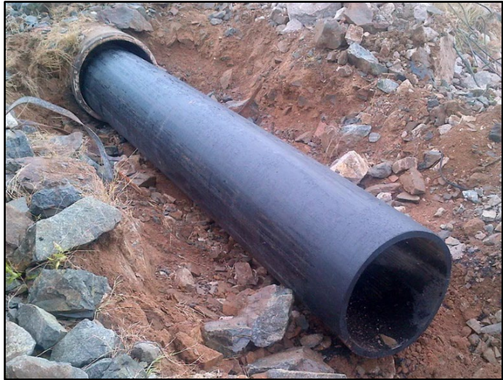
Pipe Sliplining. Image Courtesy of Downer PipeTech
