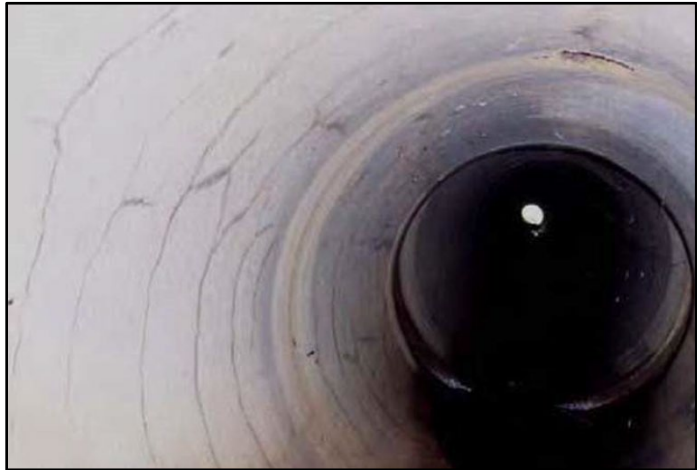
Hairline Cracking.
