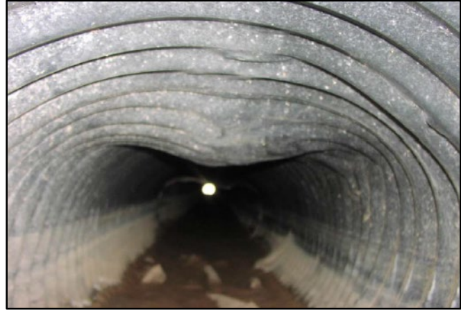
Buckling. Image Courtesy of Simpson, Gupertz & Hager
