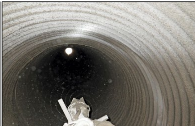
Centrifugally Installed Liner. Image Courtesy of Centi-Lining
