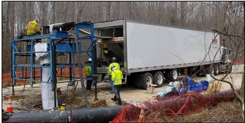
Pipe Liner Installation. Image Courtesy of Standard Pipe Services
