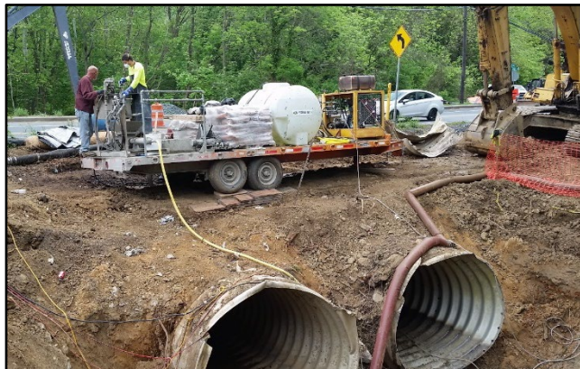
Centrifugally Installed Liner. Image Courtesy of Standard Pipe Services
