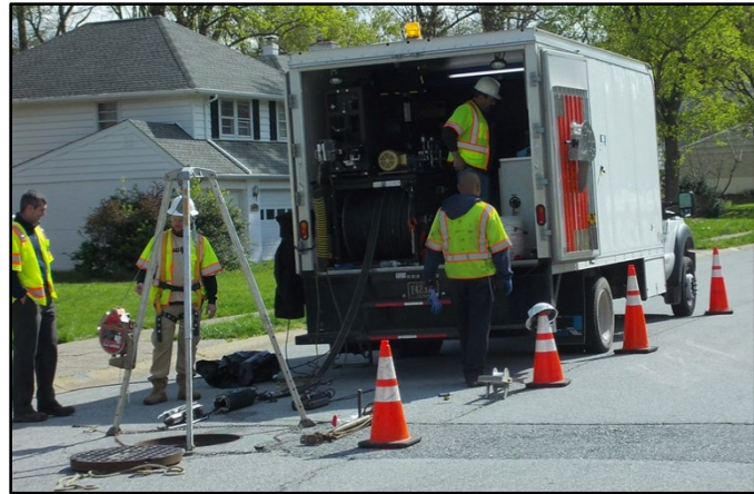
Pipe Cleaning Operation. Image Courtesy of Standard Pipe Services
