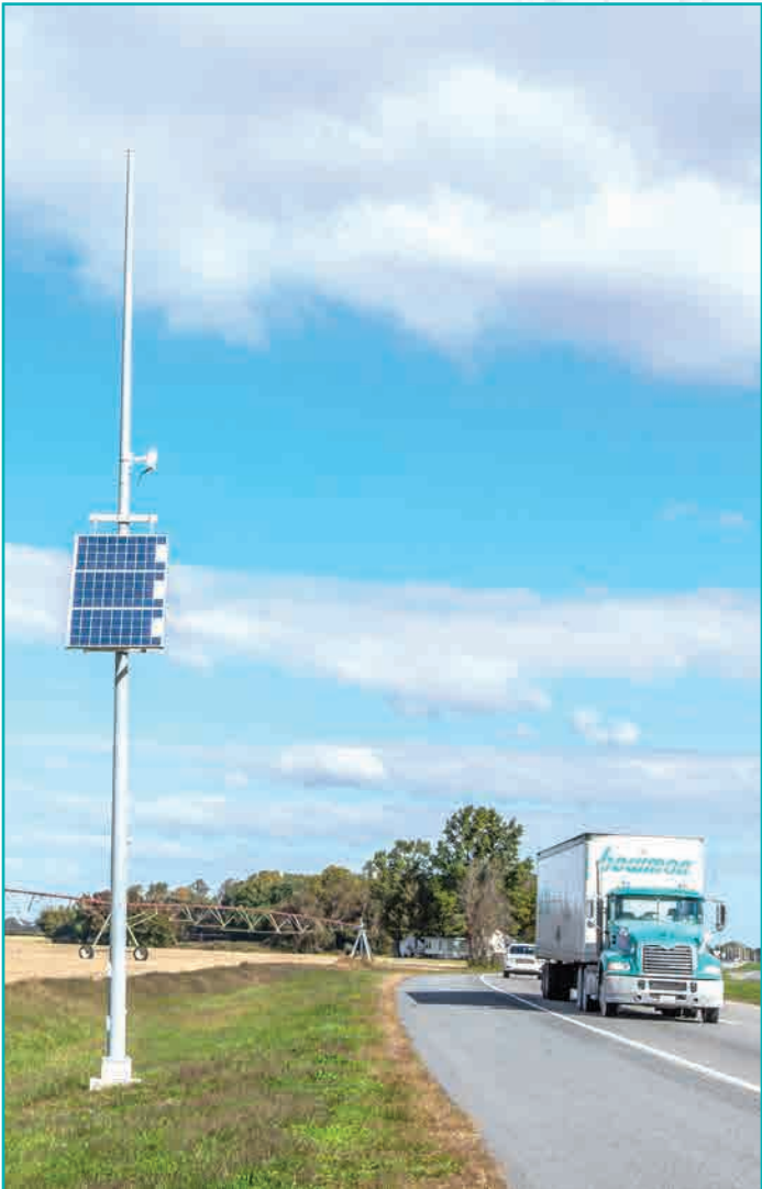
Radar traffic detection is unobtrusive, meaning out of the lanes.
