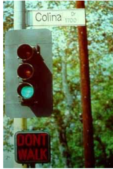
Figure 33. Traffic signals are needed to improve pedestrian crossings on some high-volume or multilane roads.
