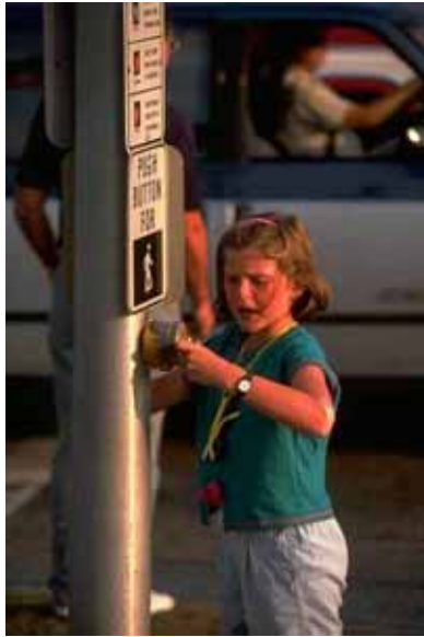
Figure 32. Pedestrian signals help accommodate pedestrian crossings on some high-volume or multilane roads.
