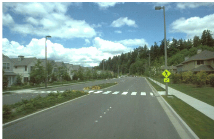
Figure 31. Raised medians and crossing islands can improve pedestrian safety on multilane roads.
