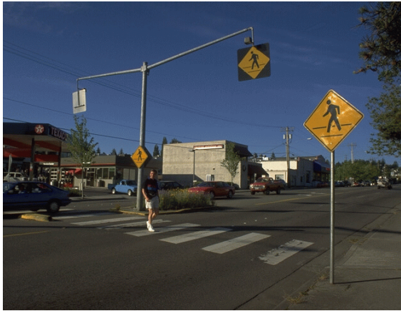
Figure 5. High visibility crossing with pedestrian crossing signs in Kirkland, WA.
