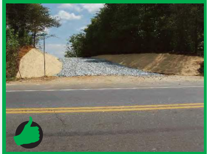
A. Stabilized Construction Entrance
