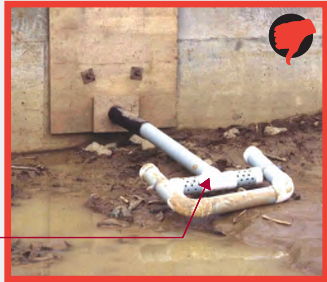
C. Skimmer Dewatering Device
