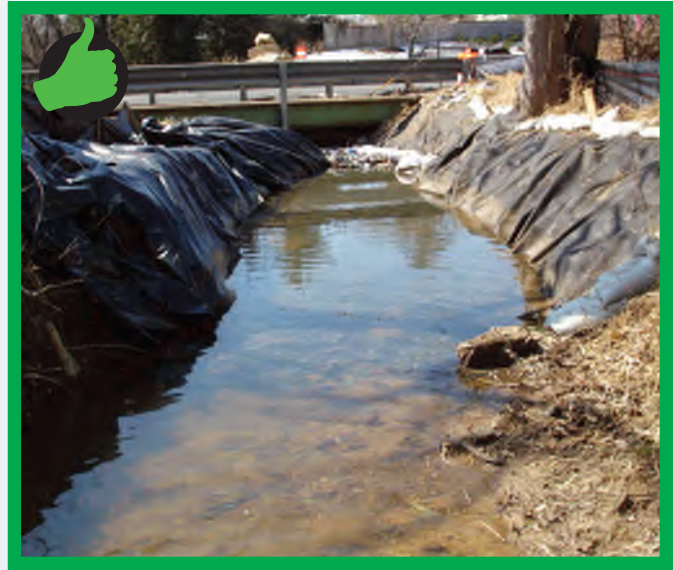
A. Geotextile-lined Diversion Channel
