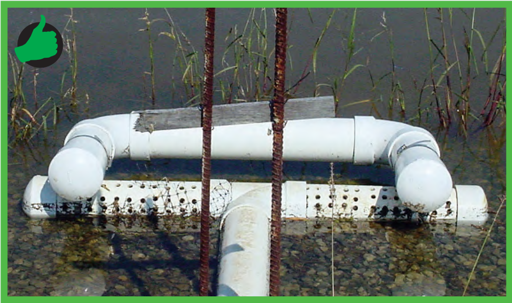
C. Skimmer Dewatering Device
