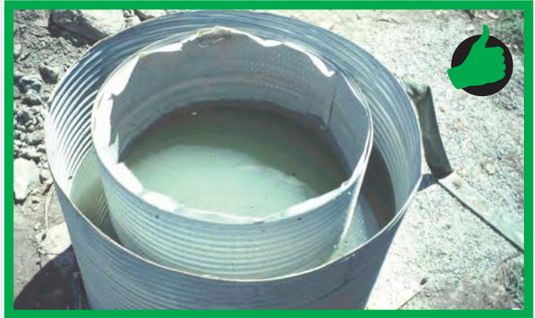
D. Portable Sediment Tank
