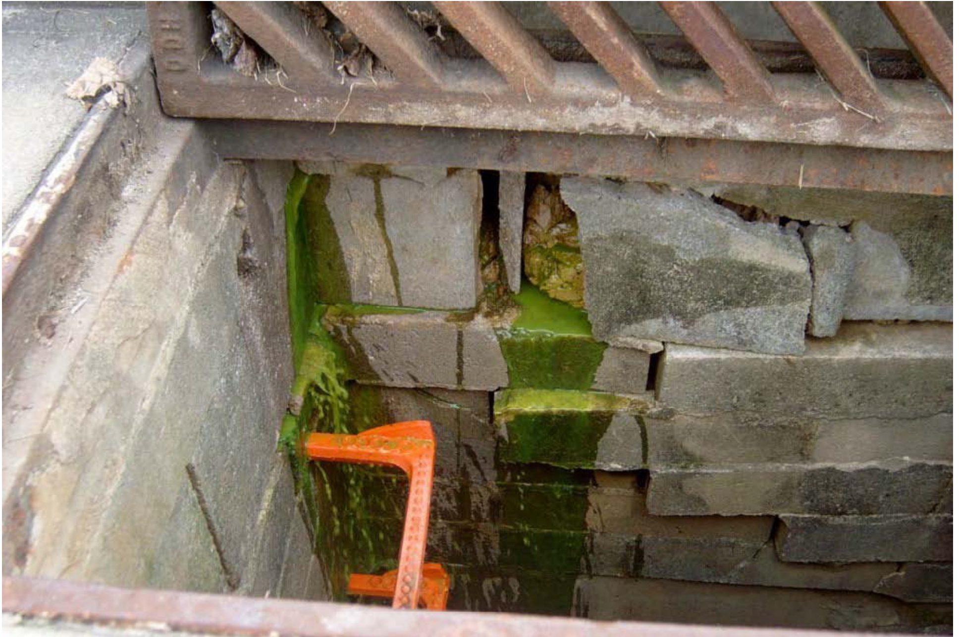
MASONRY - Displaced
