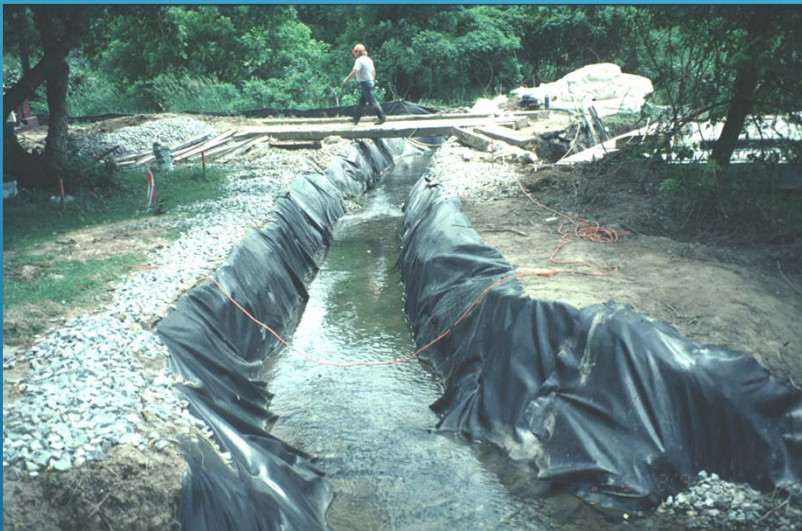
Geotextile Lined Channel Diversion (E-17)
