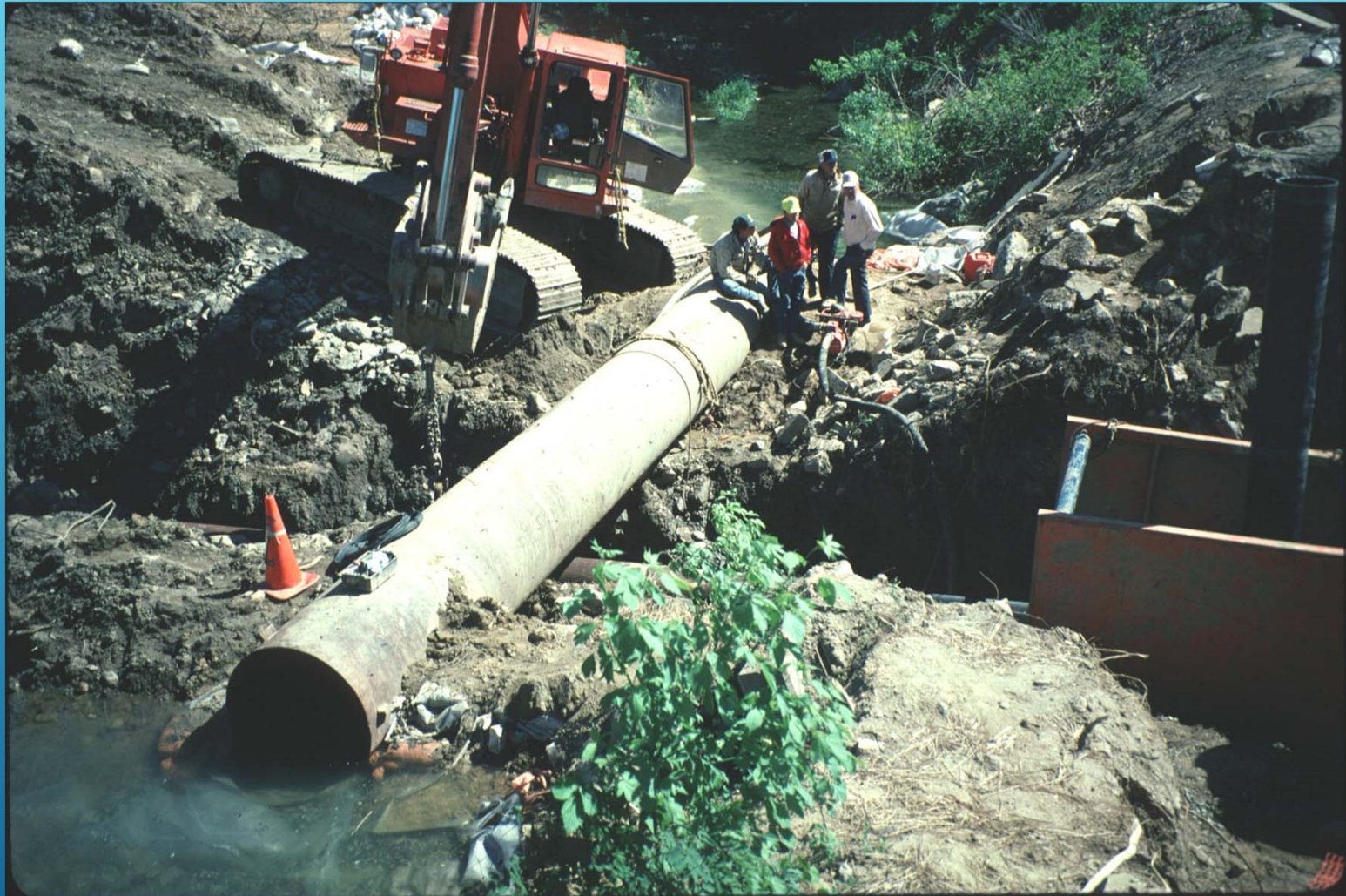
Steel Pipe As Temporary Diversion Pipe
