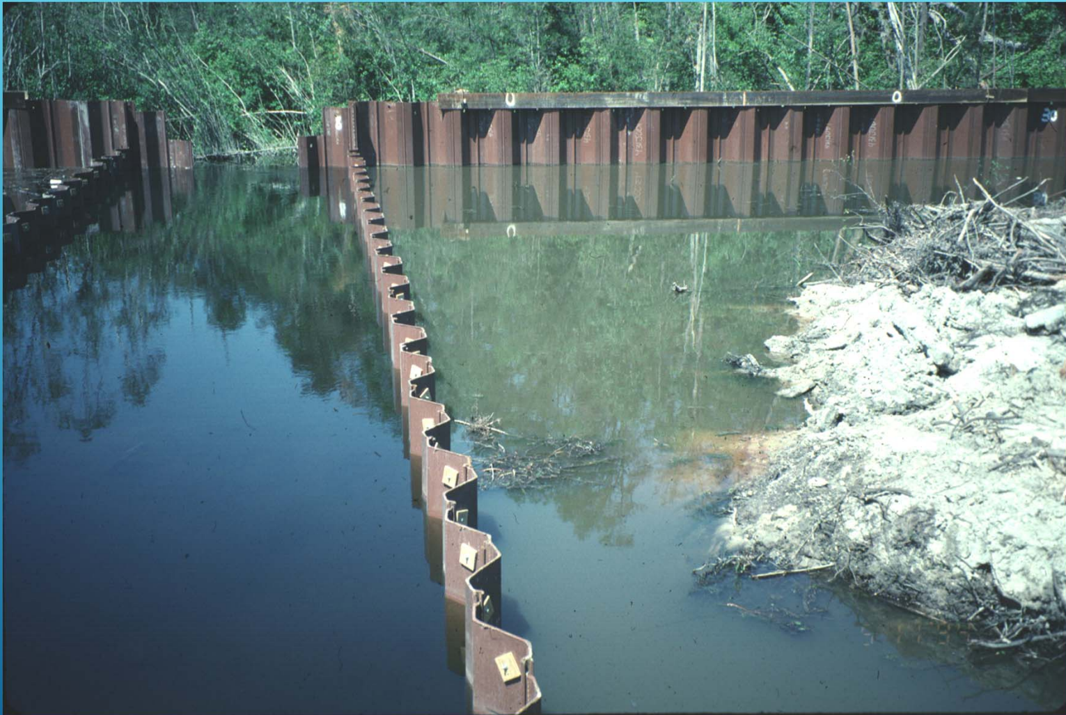
Steel Sheet Pile as Stream Diversion
