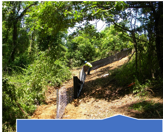
Super Silt Fence
