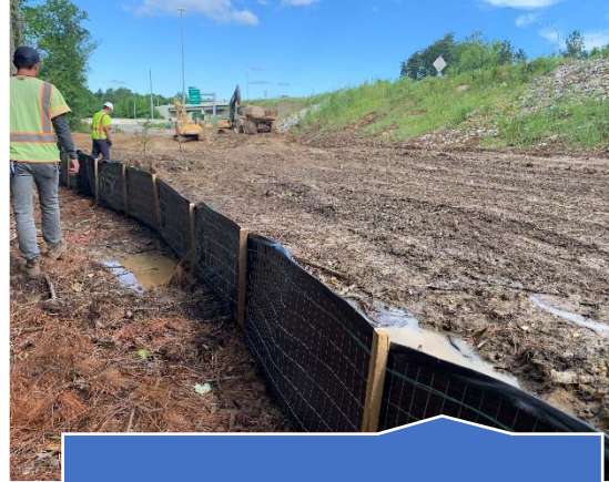
Reinforced Silt Fence
