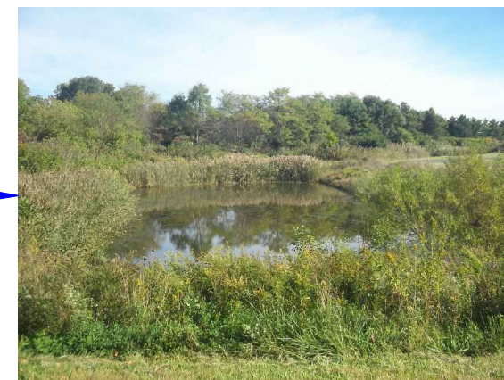
STORMWATER MANAGEMENT POND
