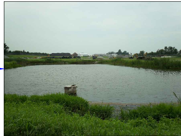
STORMWATER MGMT POND
