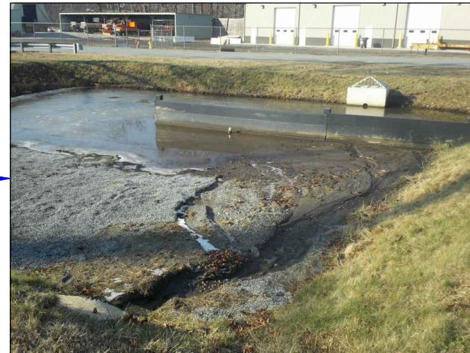
WASH PAD RETENTION POND
