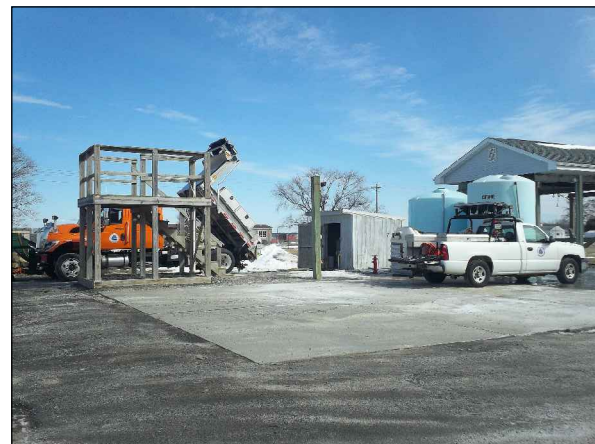
CONCRETE WASH PAD
