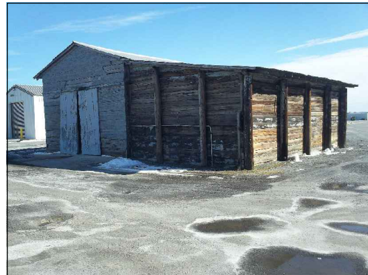
OLD WASH BUILDING
