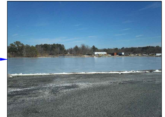
STORMWATER MGMT POND
