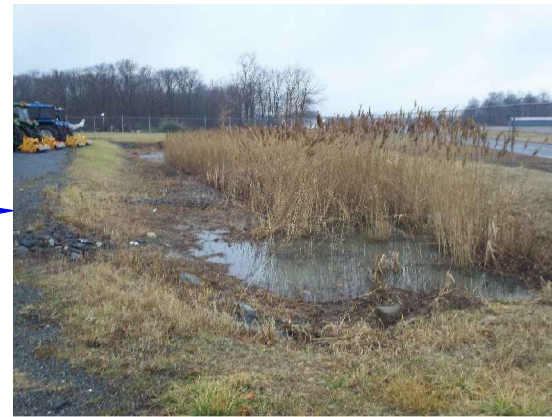
STORMWATER MGMT POND
