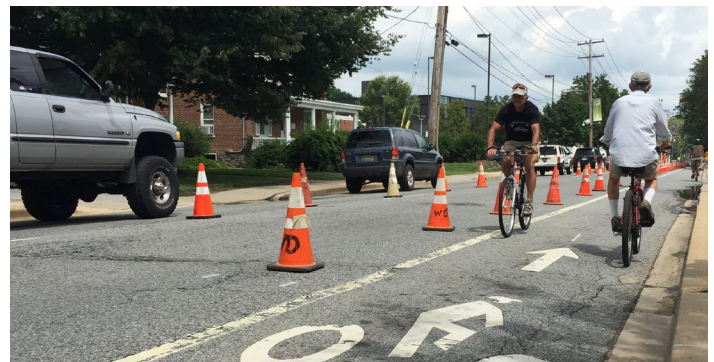
Temporary Bike Lanes on Delaware Avenue, Newark, Delaware
