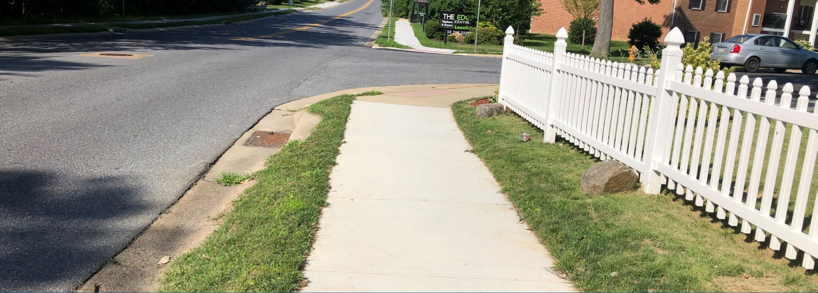
Sidewalk Link Installed through the Pedestrian Access Routes (PAR) Program
