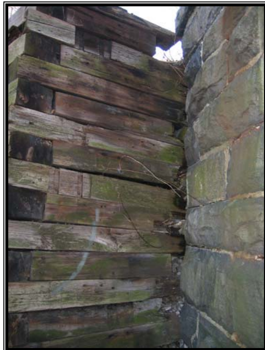
Fig. 9.8- North wing wall at east abutment
