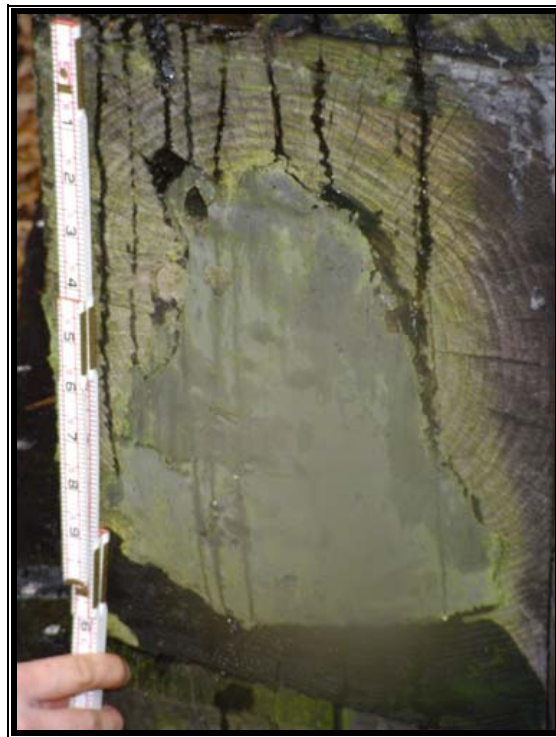
Fig. 6.4- Typical repair on abutment
