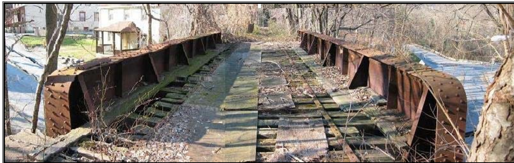
Fig. 9.4- View of superstructure from east
