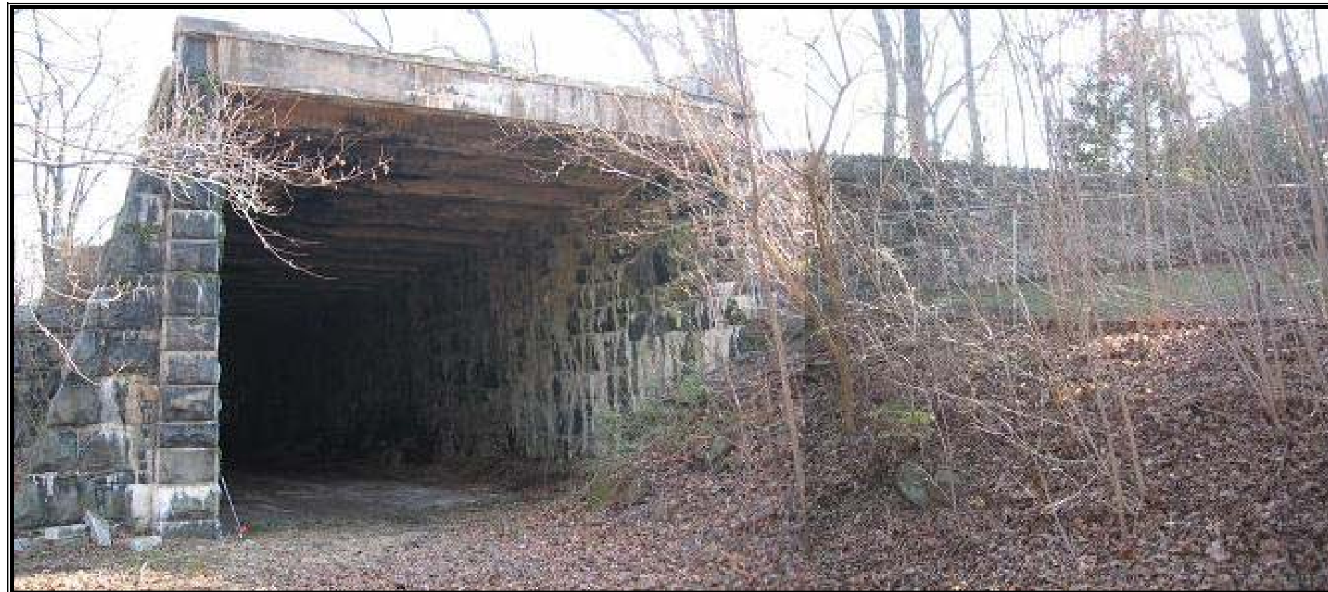
Fig. 8.1- West end of tunnel
