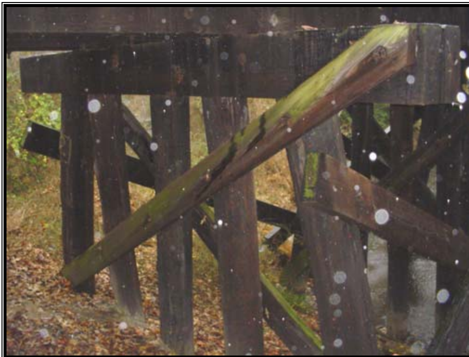
Fig. 5.1- Typical pier arrangement
