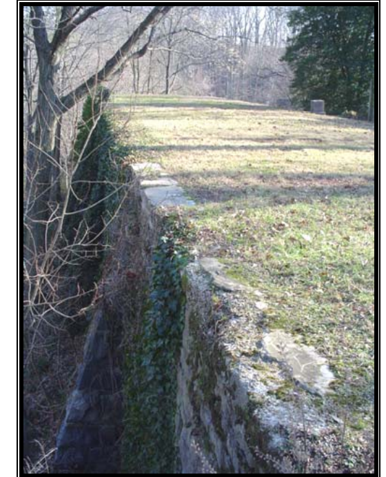
Fig. 8.4- Tunnel roof with maintained turf, view from west
