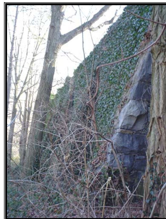
Fig. 8.6- North abutment with buttress
