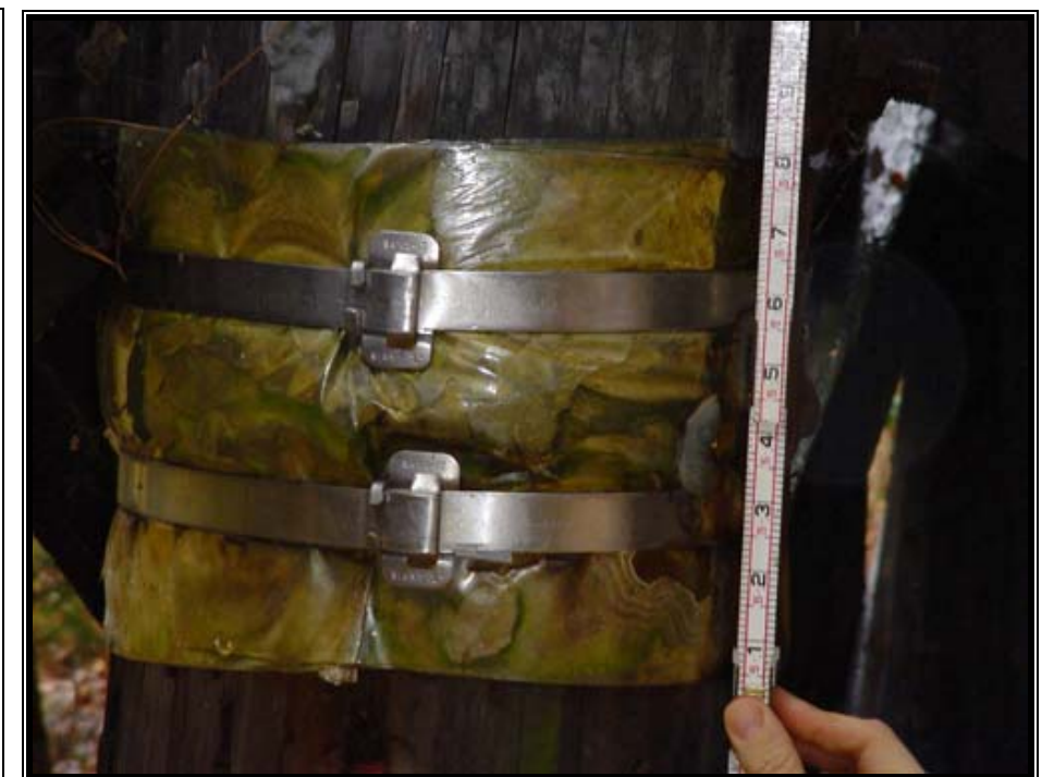
Fig. 5.3- Jacketing at pier 2
