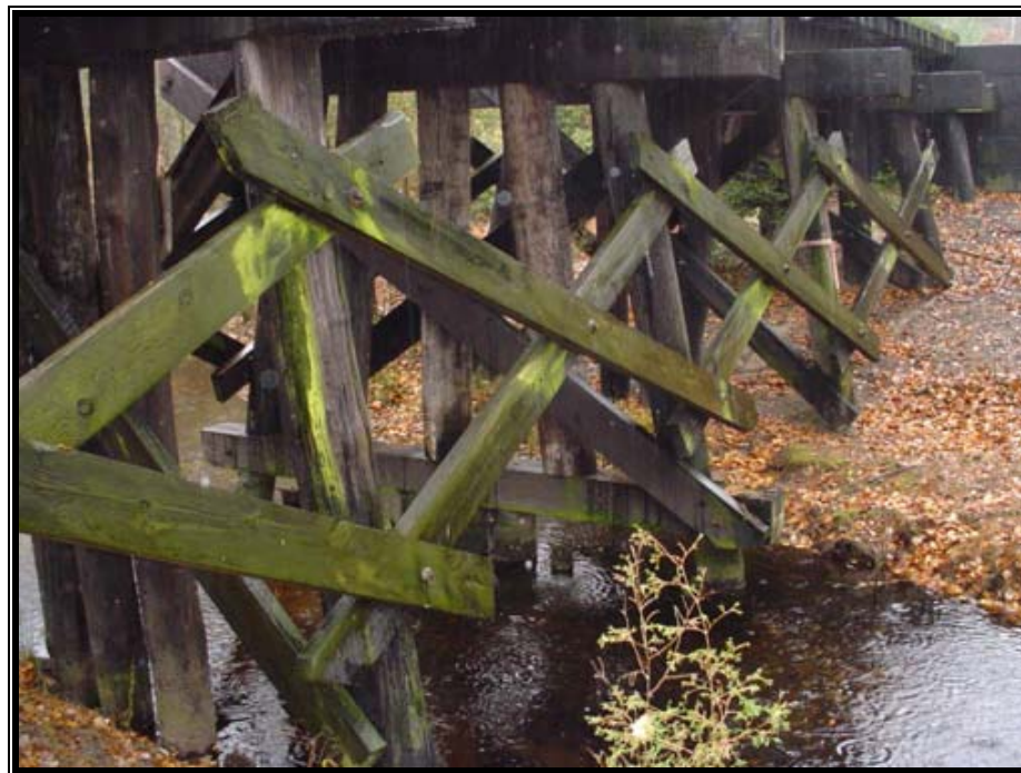
Fig. 5.4- Typical cross bracing between piers
