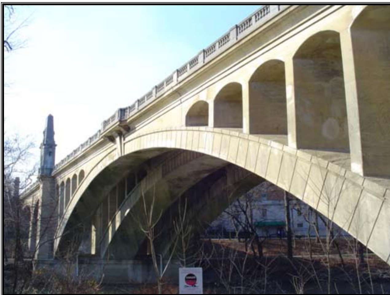
Fig. 4.1- General view of bridge over the Brandywine Creek from rail corridor
