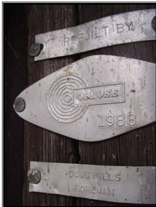
Fig. 6.7- Metal tag on pier 7, indicating when the structure was rebuilt
