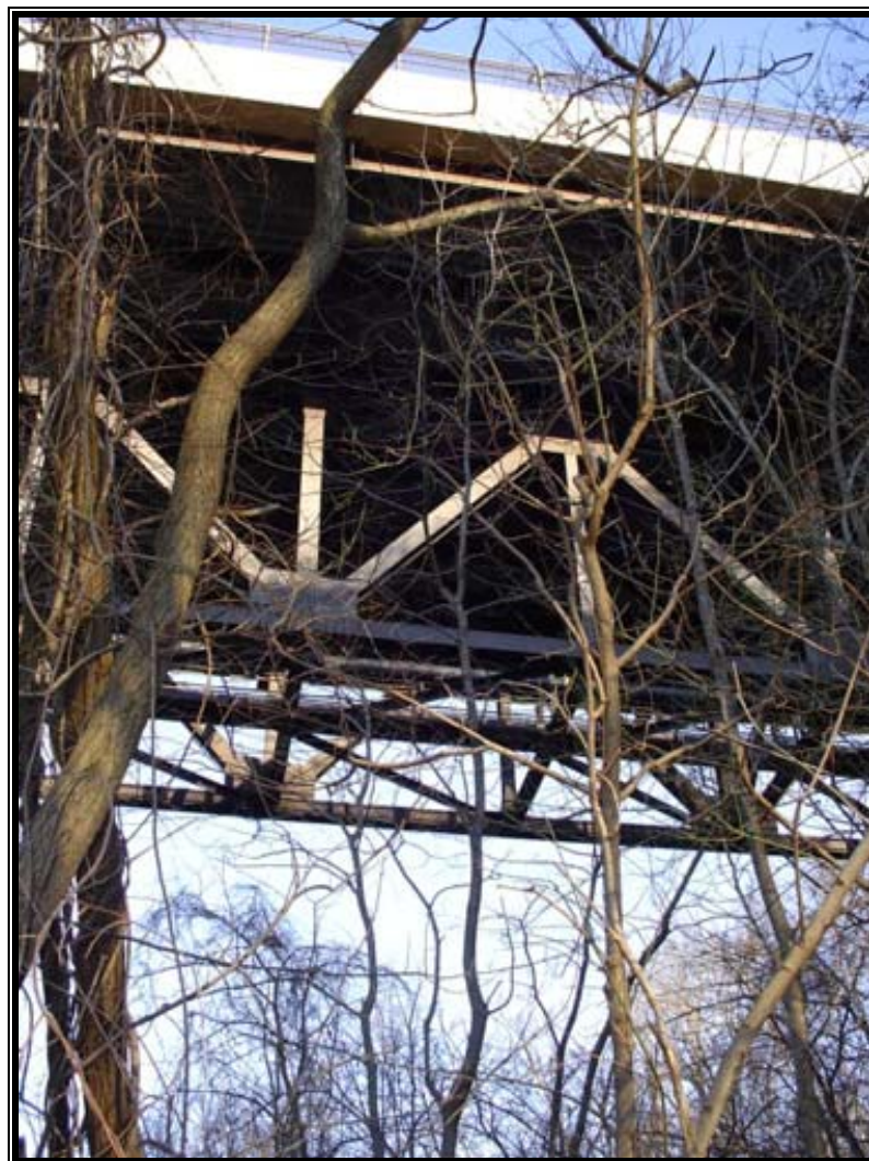
Fig. 1.1- View from below at the northern terminus of the existing trail
