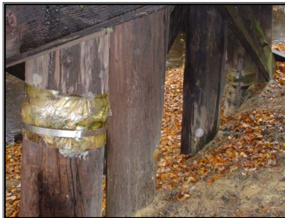
Fig. 5.2- Jacketing around pile 1 at pier 5
