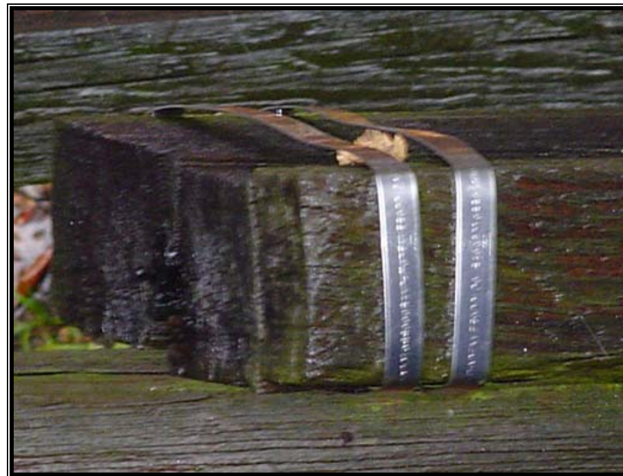
Fig. 5.5- Banding on cross bracing at pier 4
