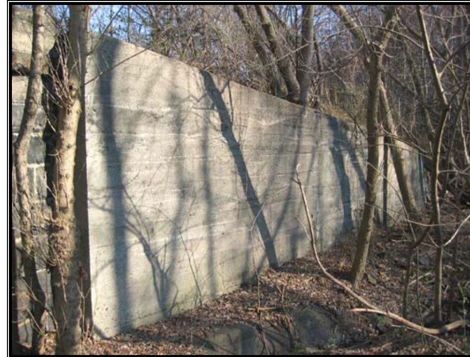
Fig. 9.10- South wing wall
