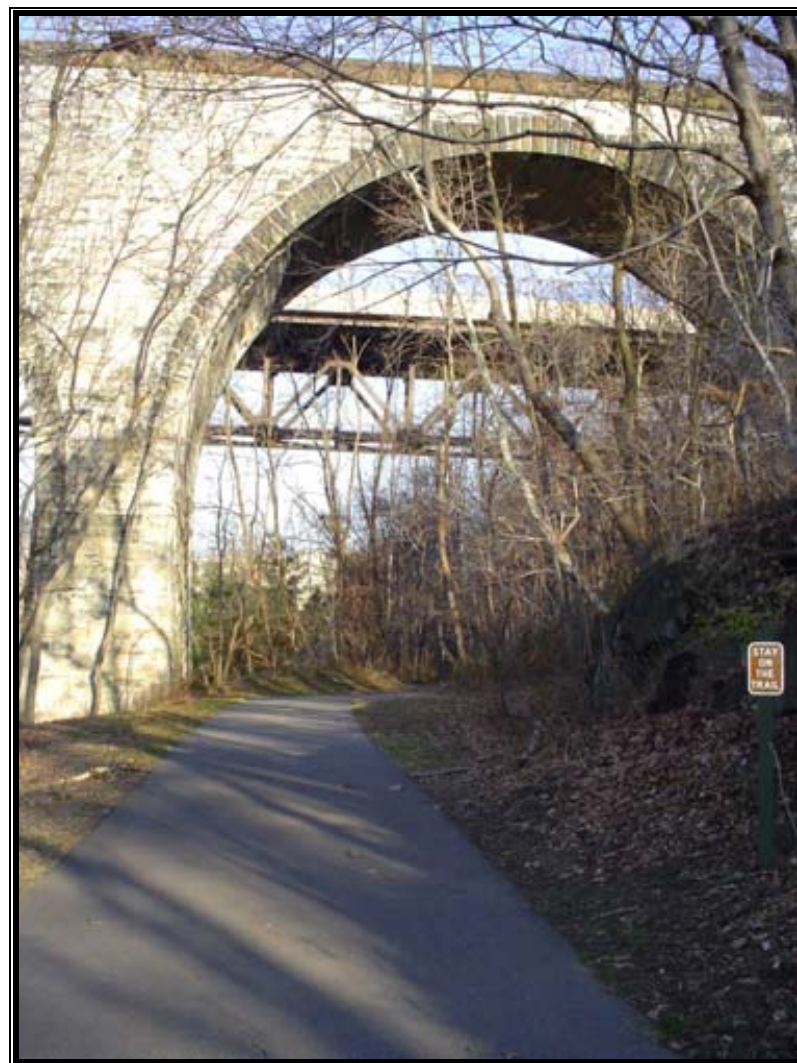
Fig. 2.1- View of stone railroad bridge over the northern terminus of the existing trail
