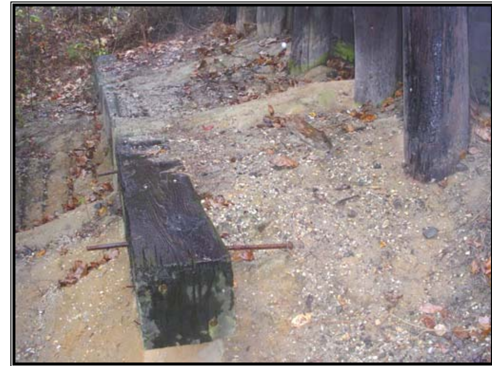
Fig. 6.6- Timber used for slope protection
