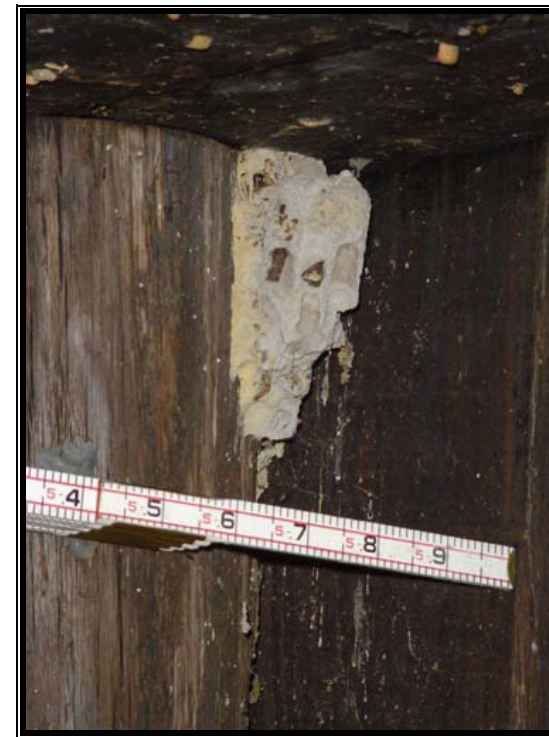
Fig. 6.5- Evidence of insect infestation
