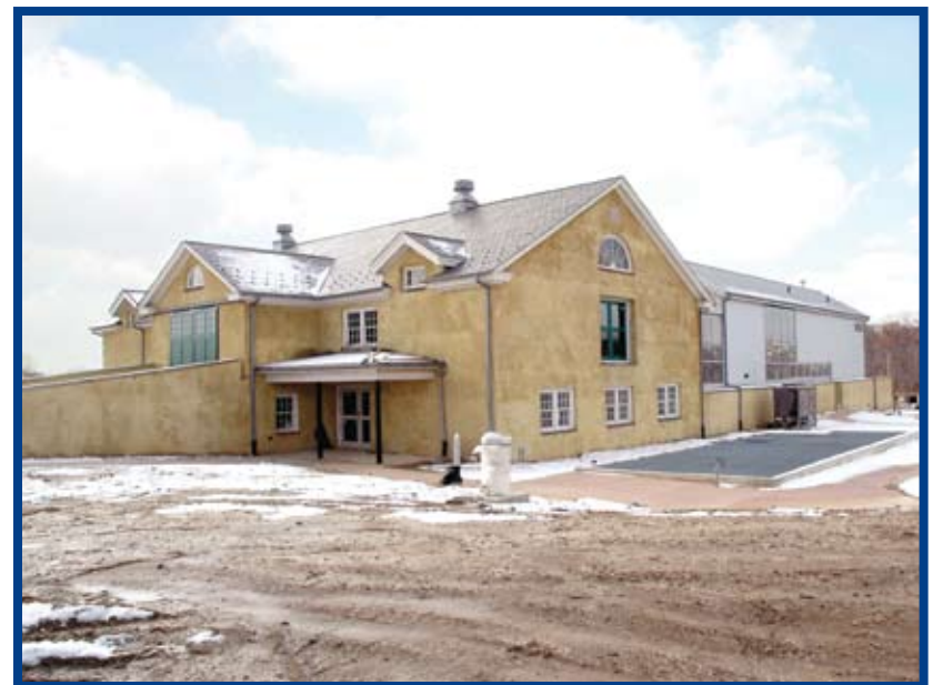
Example of a current project: BlueBall Dairy Barn renovations in progress.
