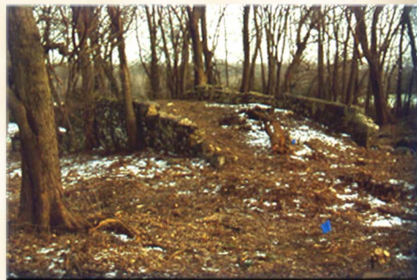
Animals and wagons would have used this ramp to enter the bank barn.
