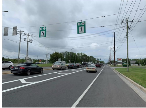
US Route 9 approaching signal at Plantation Road Connector
