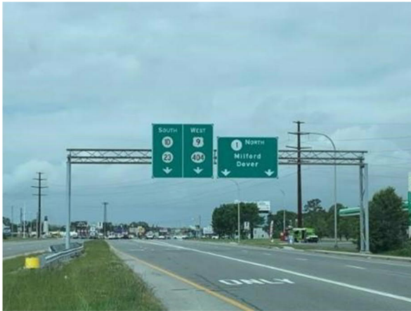
Northbound SR 1 left turn lane signing
