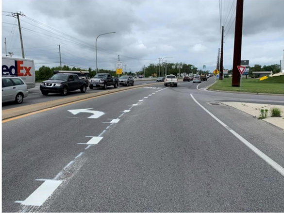
US Route 9 after turning left from SR 1
