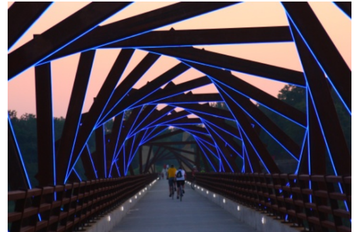
High Trestle Trail Bridge, Madrid, Iowa Source: http://iowagirlonthego.com/2011/09/04/high-trestle-trail/
