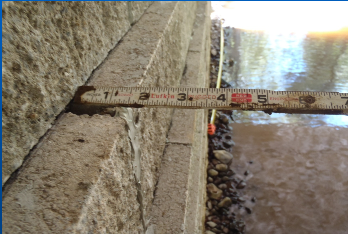
East Abutment – Uneven Battering or Bulging (~8 Feet Below Girders)
