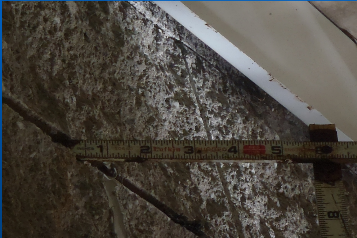
East Abutment – ¾" Wide Joint Gap in 2nd Row from Top (Looking Up)
