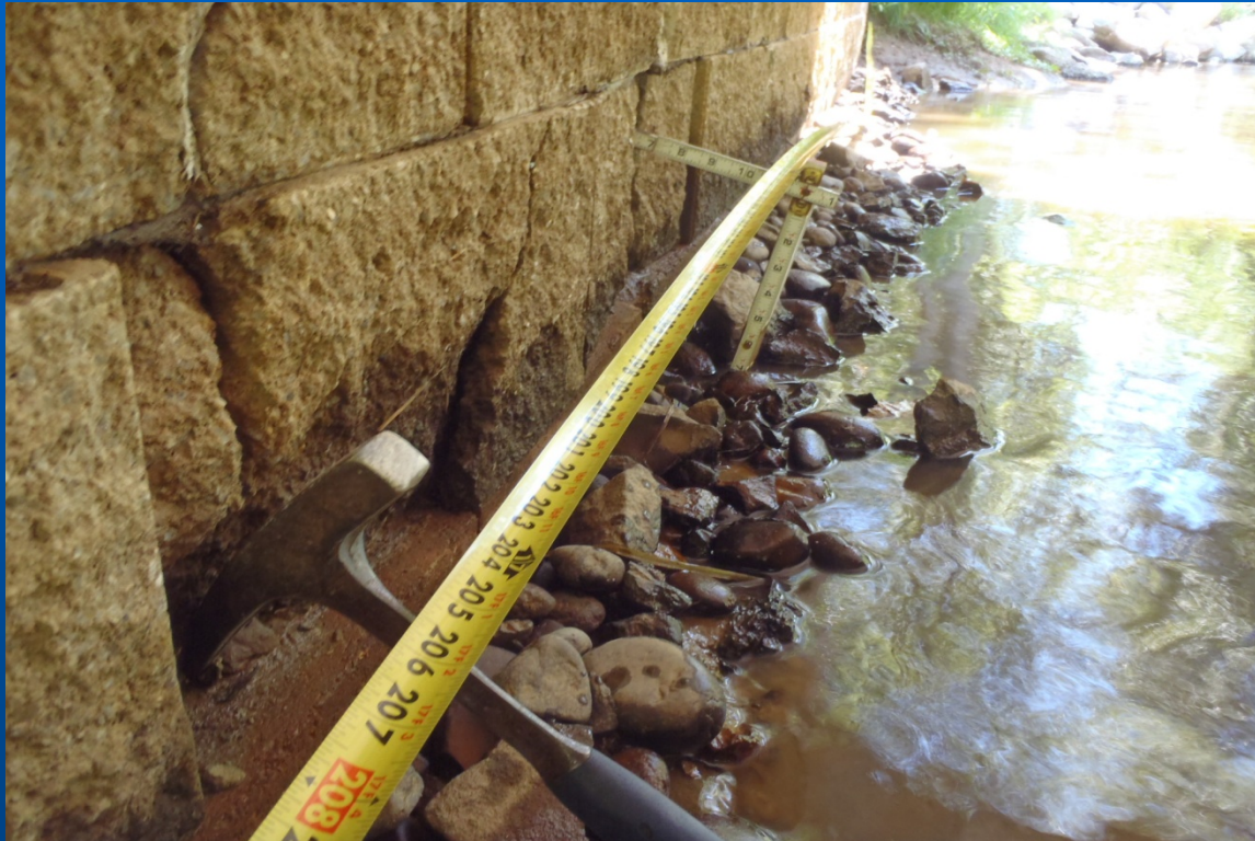
East Abutment with Broken Blocks (Looking South)
