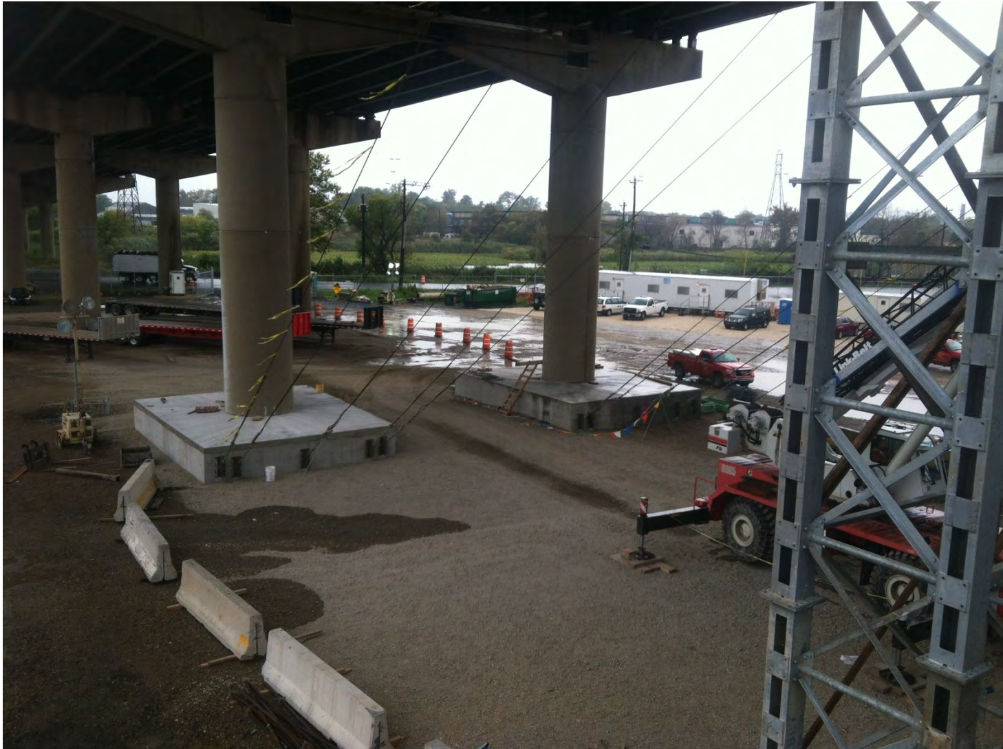
Completed underpinning and longitudinal bracing
