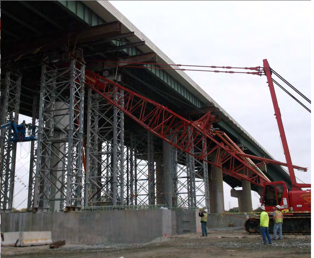
Removing Columns
