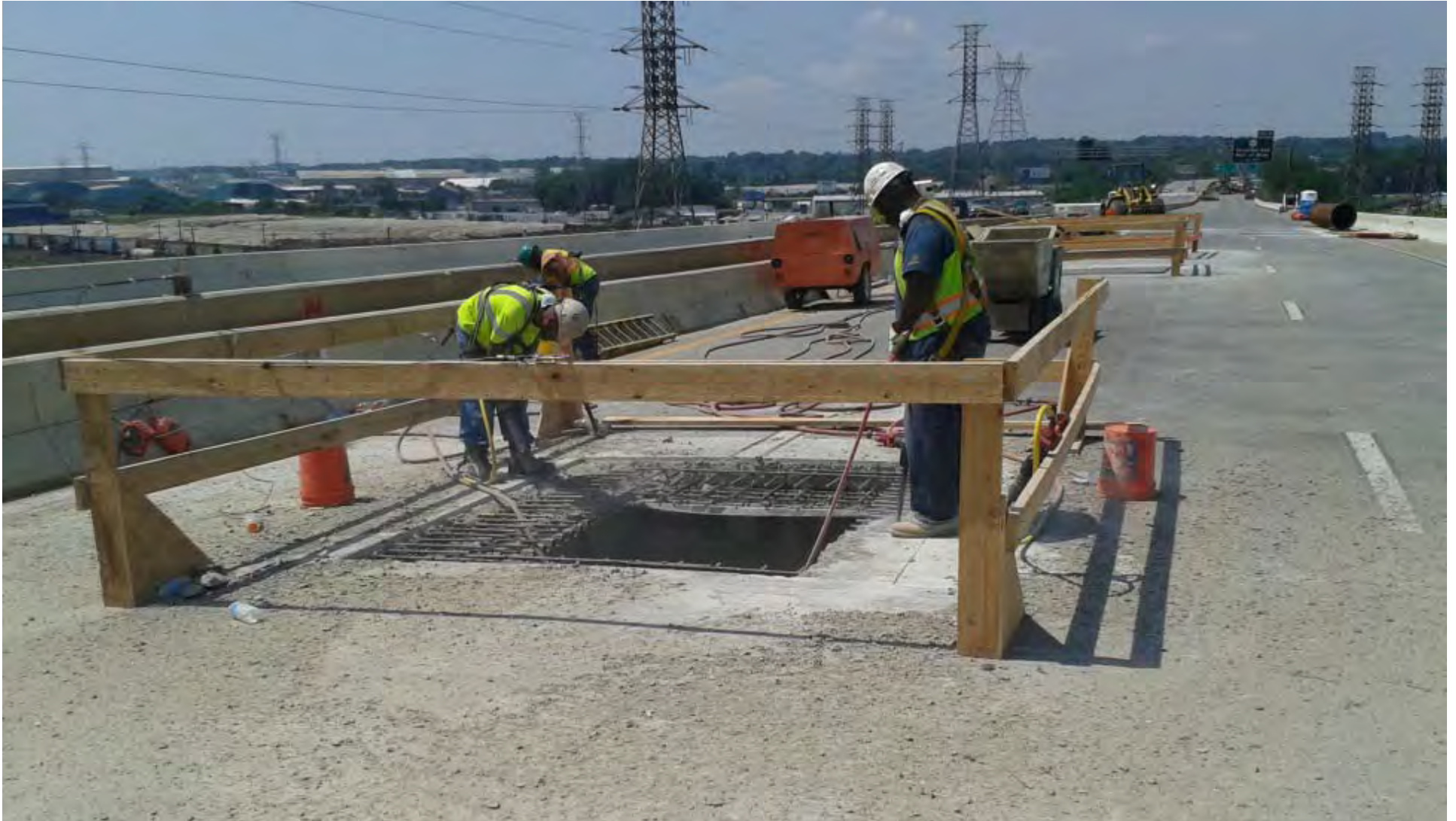
Access Holes in Bridge Deck for Placement of Drilled Shaft Rebar
