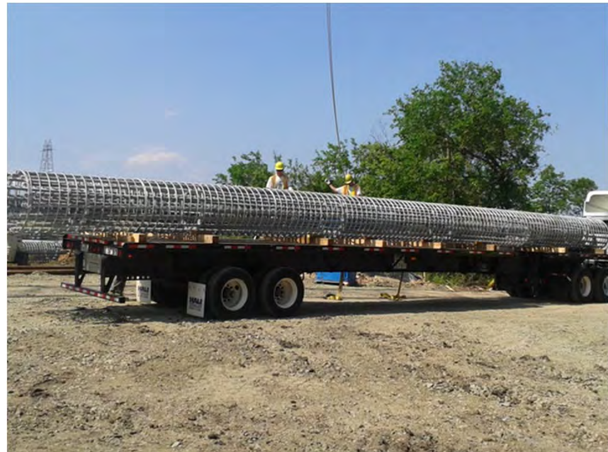
Rebar Cage from Tappan Zee 6/16/2014
