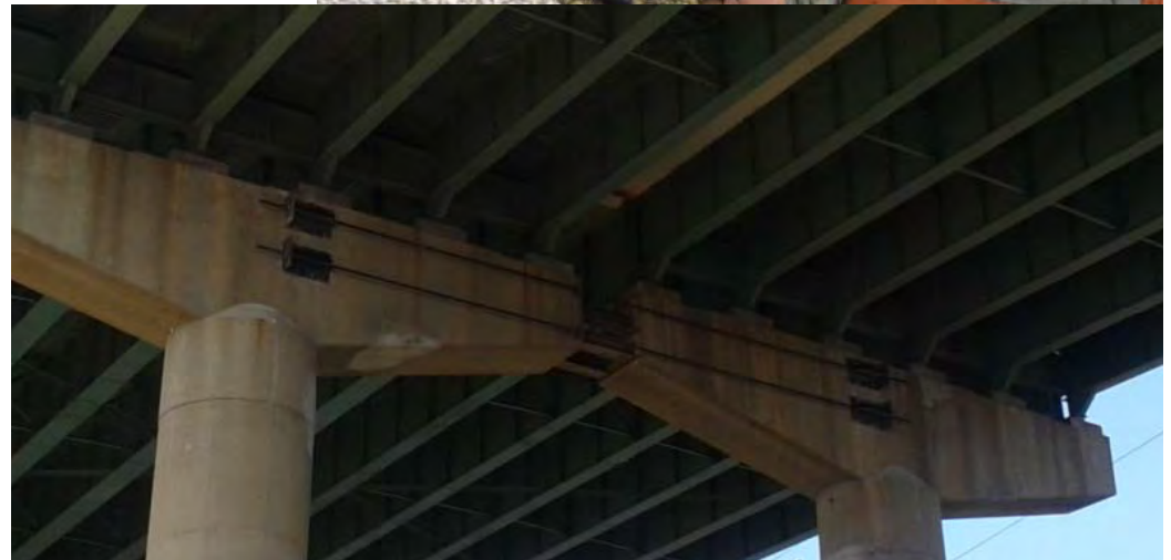
Pier Ties Installed
