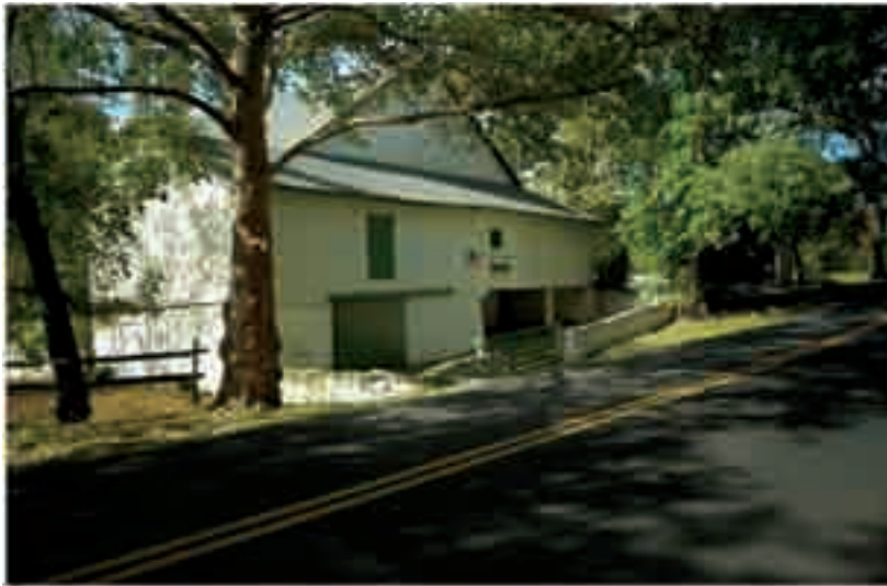
25. Centerville Road near Hillside Road
