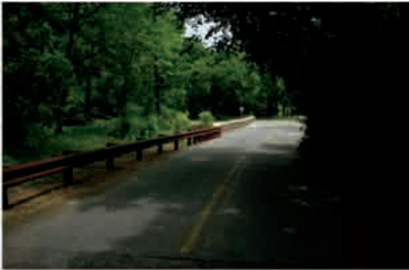
62. Sharpless Road Bridge
