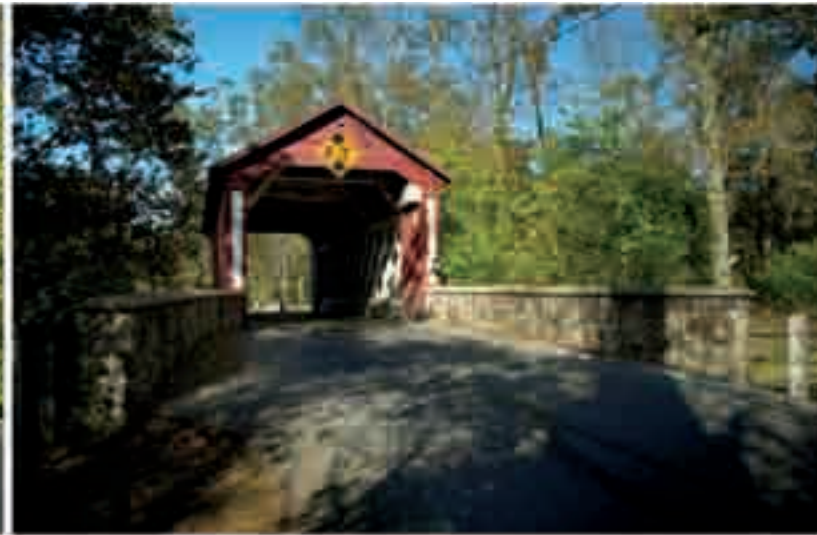
6. Brackenville Road (Ashland Bridge)
