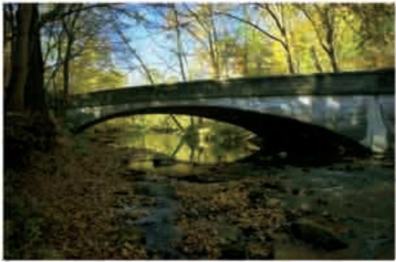
1. Mt Cuba Road (Creek Road) Bridge
