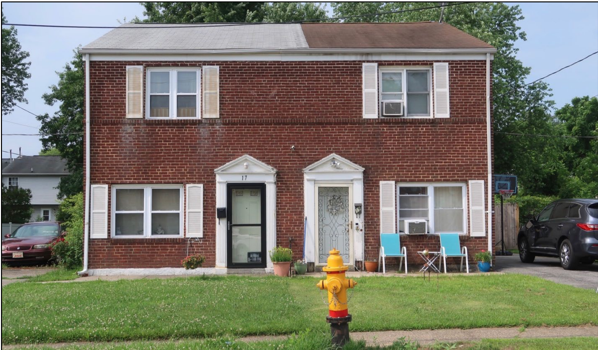
Figure 82. View of a semi-detached, two-family home in Rose Hill Gardens showing the brick veneer siding, brick belt course, shutters, and triangular pedimented door surrounds. (Center for Historic Architecture and Design, 2021)
