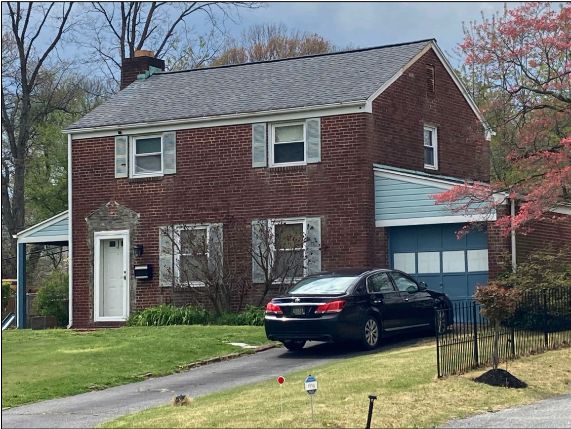
Figure 121. Example of a two-story, brick veneered “Colonial” constructed in Swanwyck during the 1940s. (Center for Historic Architecture and Design, 2022)
