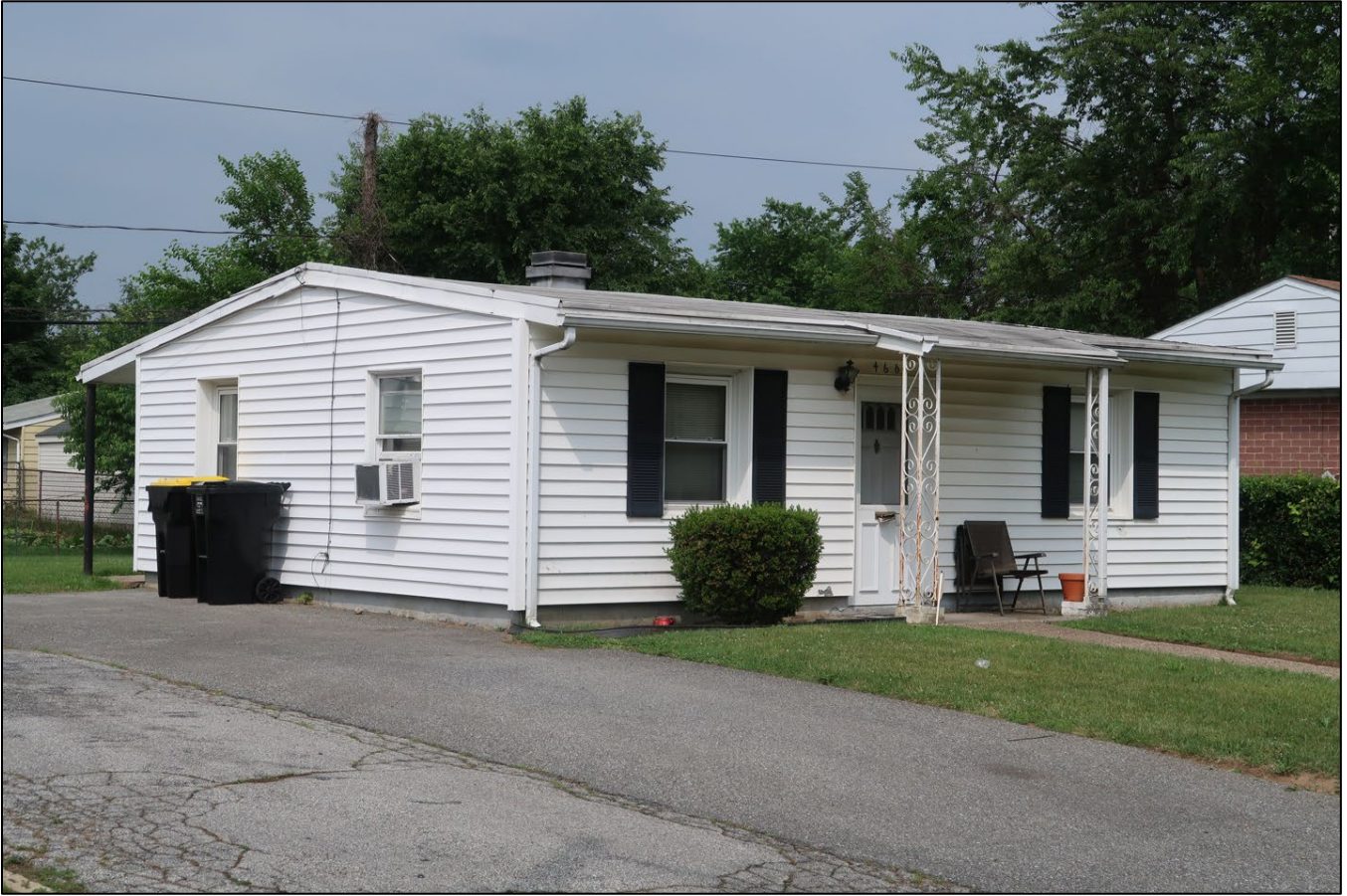
Figure 88. Example of a three-bay ranch form house in Dunleith. This dwelling has been slightly modified with newer vinyl siding and porch supports. (Center for Historic Architecture and Design, 2021)
