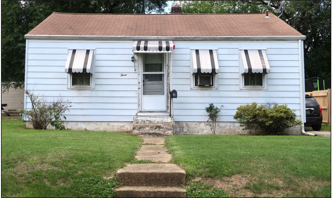
Figure 62. An example of a four-bay, Minimal Traditional ranch house. This form and size of house was typical of designs that complied with early FHA guidelines. (Center for Historic Architecture and Design, 2021)
