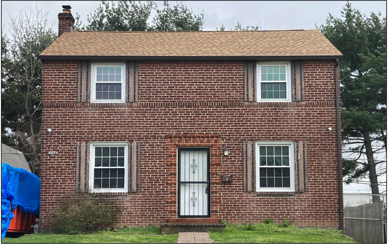
Figure 107. Example of a two-story, brick veneered "Colonial" dwelling in Collins Park. (Center for Historic Architecture and Design, 2022)
