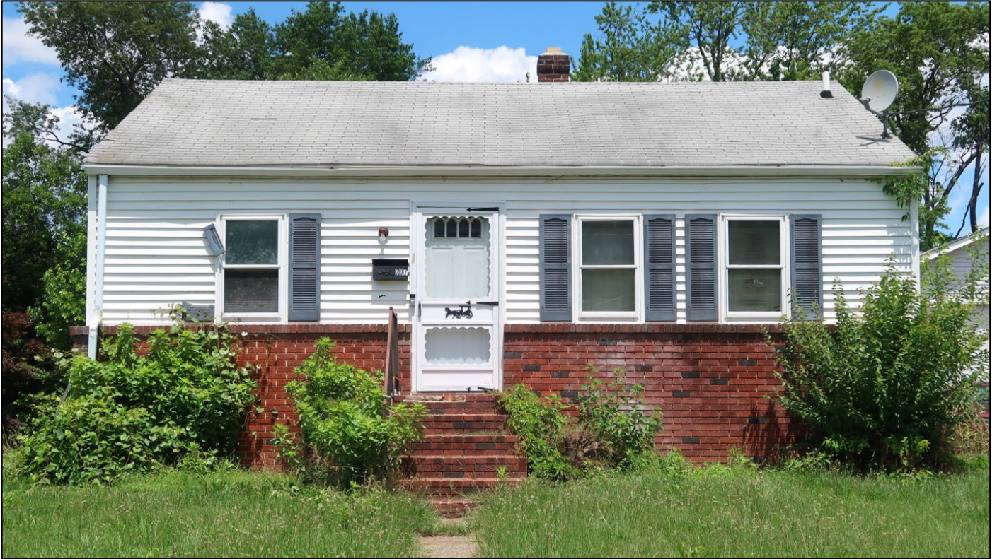
Figure 64. An example of the four-bay ranch with Early American detailing including brick veneer, louvered shutters, and scallop-edge screen door replete with horse and carriage silhouette. (Center for Historic Architecture and Design, 2021)
