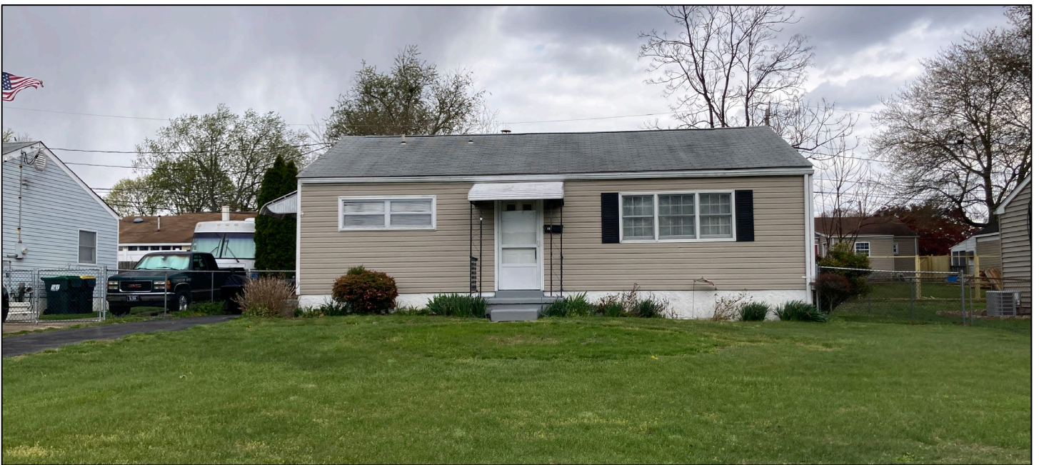
Figure 131. Example of a three-bay ranch house in Castle Hills. (Center for Historic Architecture and Design, 2022)
