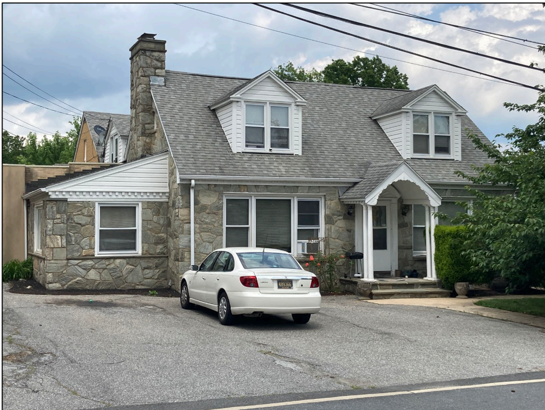
Figure 47. Example of a stone masonry house on Rizzo Avenue. (Center for Historic Architecture and Design, 2022)
