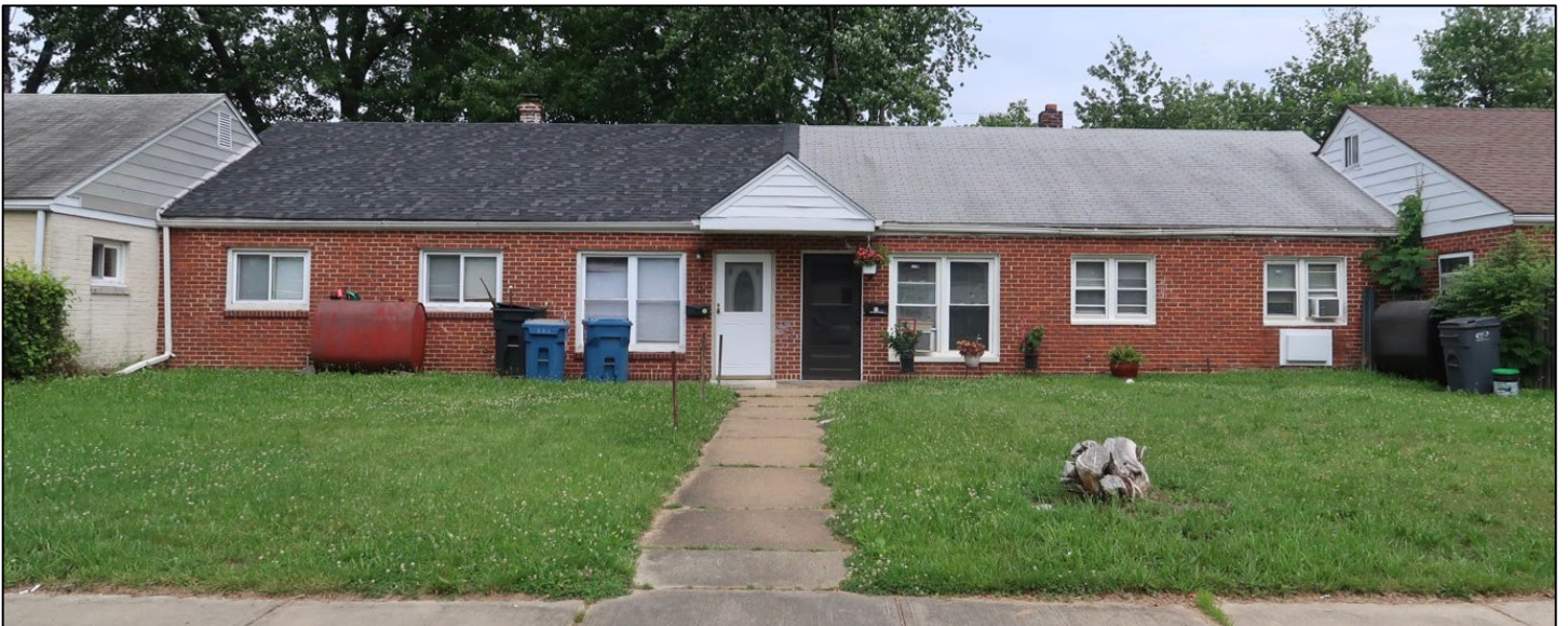
Figure 59. Example of two interior units, with the original porch overhang and shared walkway to the two separate front doors. Note the interior units are set back from the two units flanking either side. (Center for Historic Architecture and Design, 2021)
