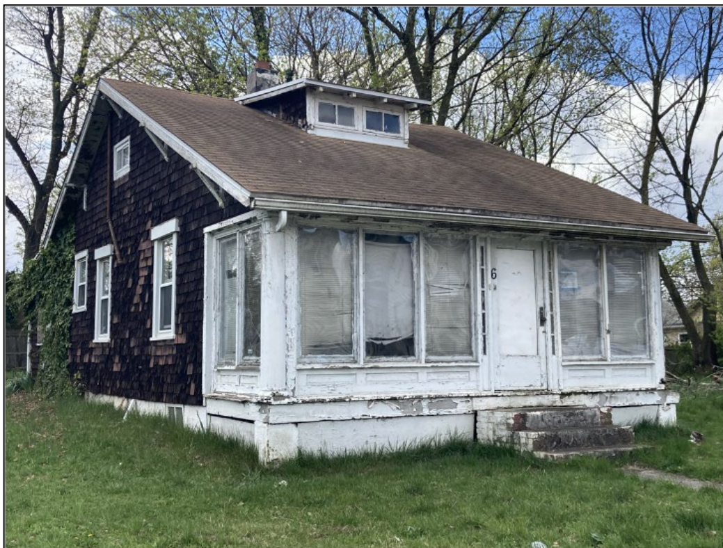
Figure 21. Example of an early-twentieth century bungalow in Hamilton Park; this dwelling retains many of its original exterior materials including wooden shingle cladding, eave brackets, exposed rafter tails, and porch columns. (Center for Historic Architecture and Design, 2022)
