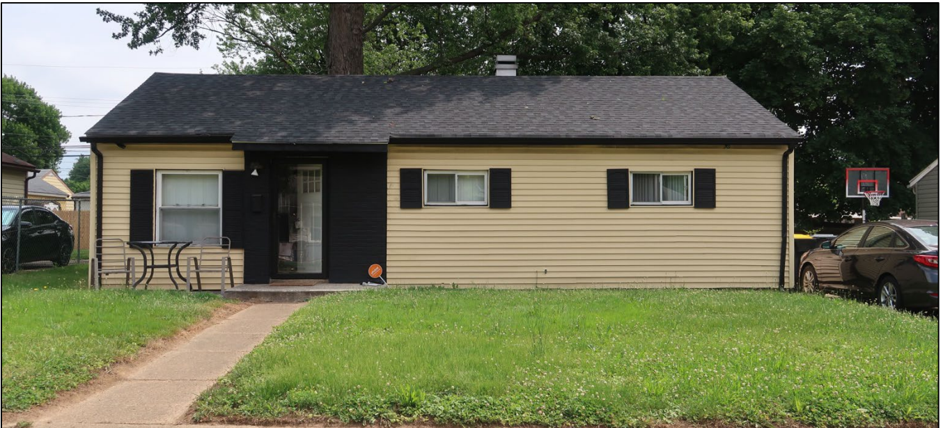
Figure 99. Example of a four-bay, side-gabled ranch house. This was the dominant form constructed in Section 1 of Garfield Park. Note the original fenestration, as well as the brick veneer (now painted black) around the door. (Center for Historic Architecture and Design, 2021)
