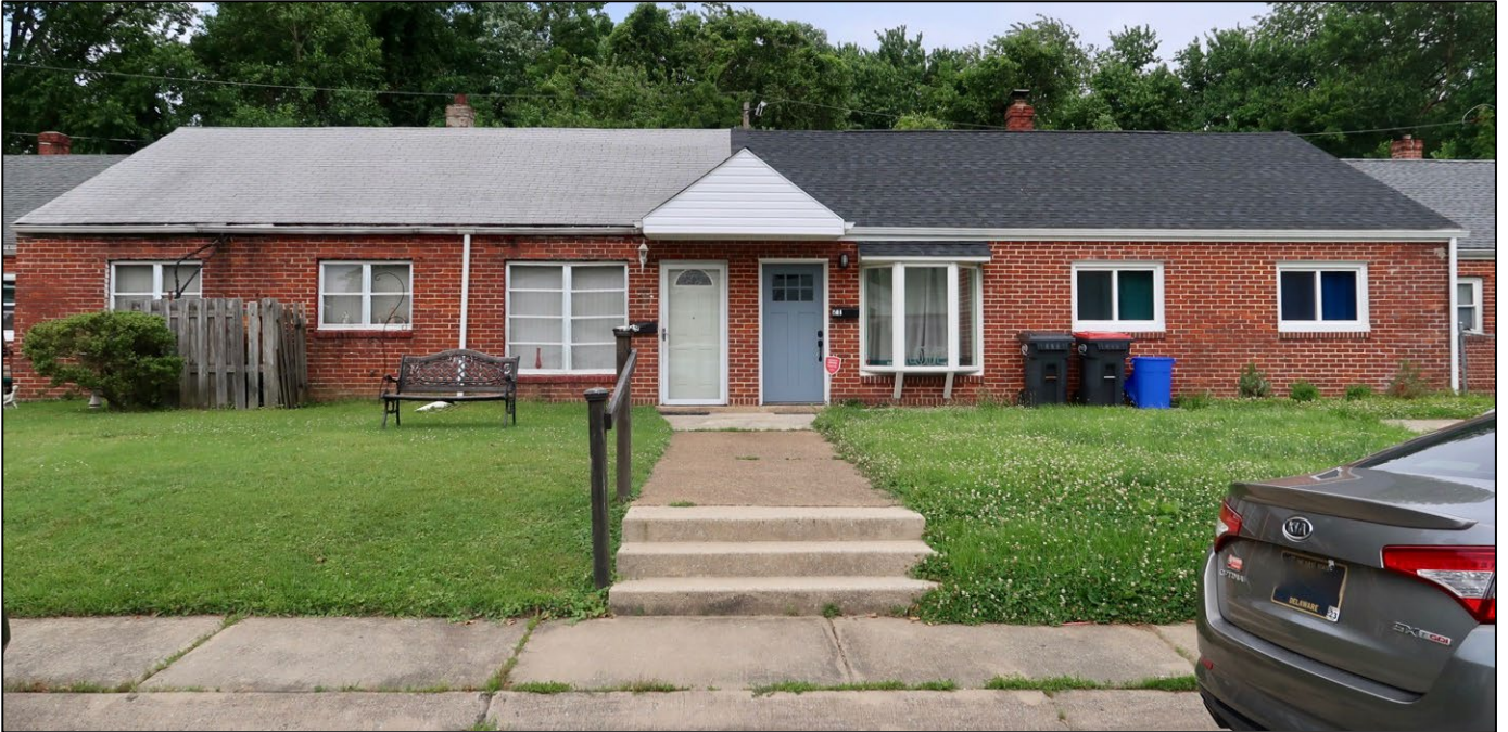
Figure 60. Example of two interior units, with the original porch overhang and shared walkway to the two separate front doors. Note the interior units are set forward from the two units flanking either side. (Center for Historic Architecture and Design, 2021)
