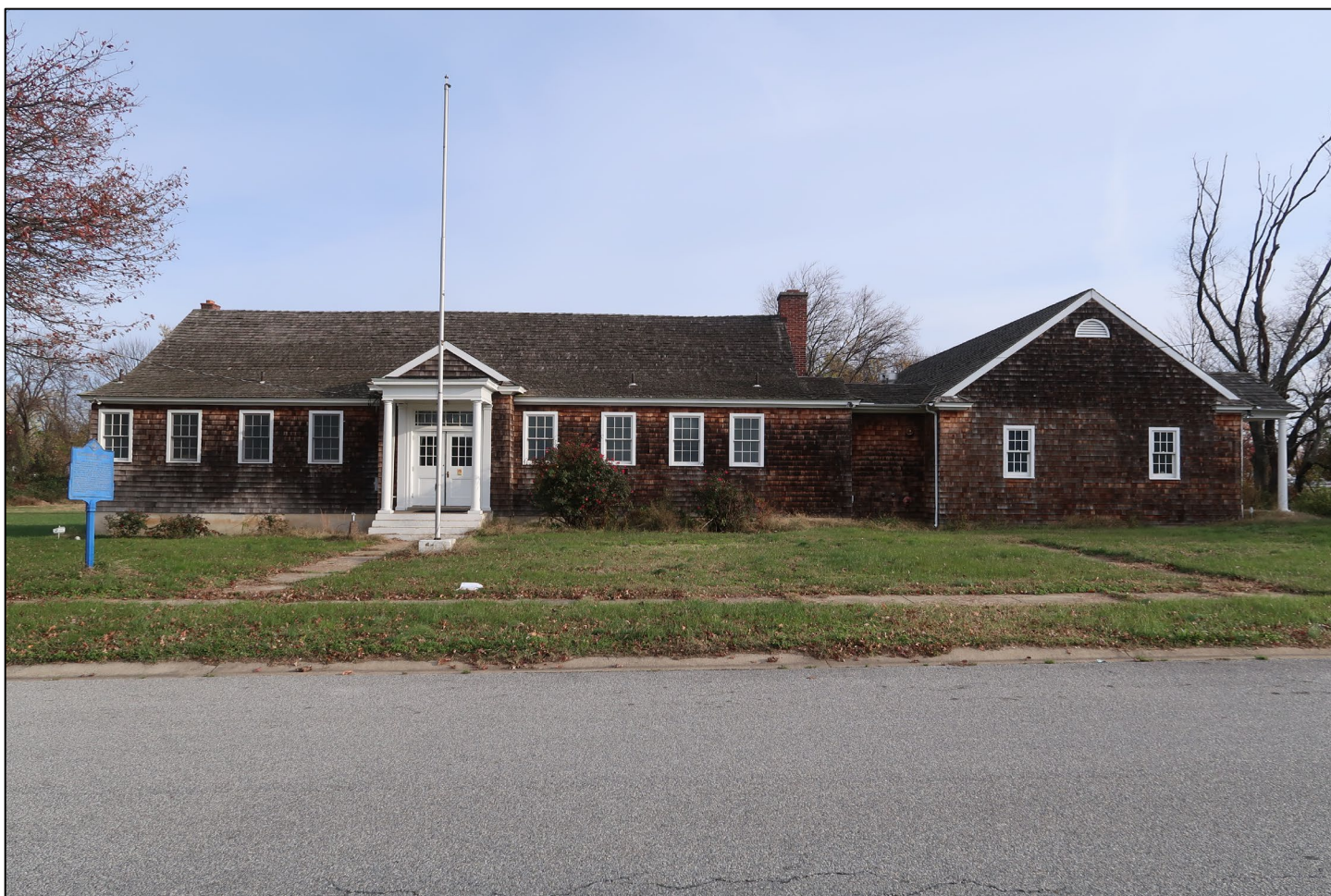
Figure 25. Buttonwood School, built in 1926 (and later expanded) as part of the Pierre S. du Pont-funded school rebuilding program through the Service Citizens of Delaware. (Center for Historic Architecture and Design, December 2020)
