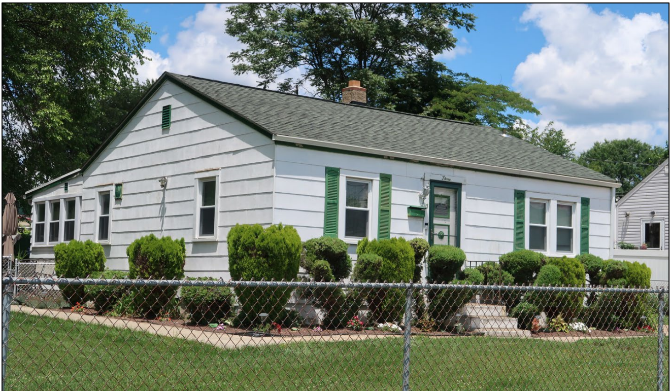
Figure 63. Above is a three-bay, Minimal Traditional ranch house. Instead of having four bays, two windows are combined into a single window feature. Both the three- and four-bay ranches have 780 square feet of living space. (Center for Historic Architecture and Design, 2021)
