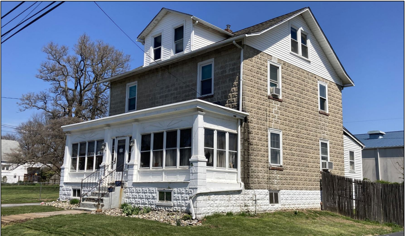
Figure 33. Example of an early-twentieth century, two-story, rusticated concrete block dwelling in Minquadale. (Center for Historic Architecture and Design)
