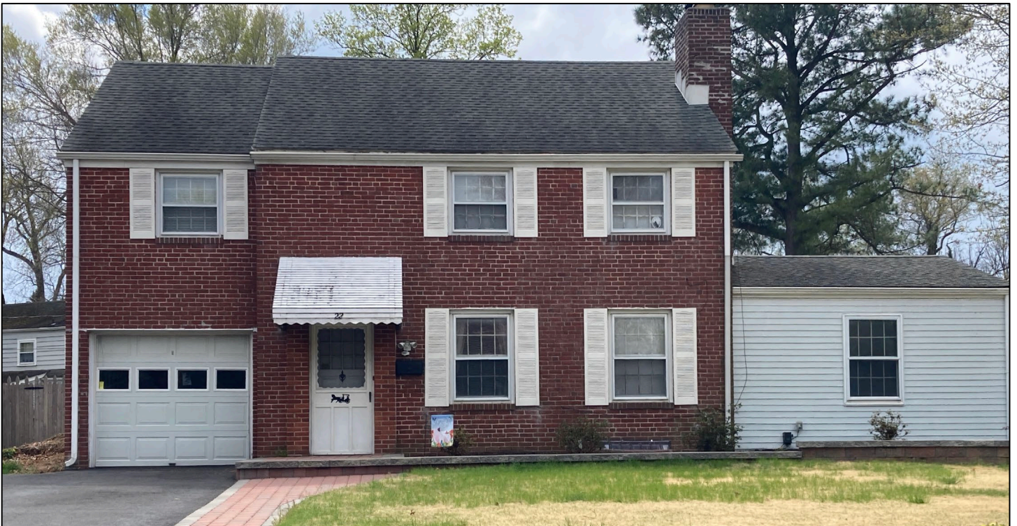
Figure 120. Example of a two-story, brick veneered "Colonial" constructed in Swanwyck during the 1940s. (Center for Historic Architecture and Design, 2022)
