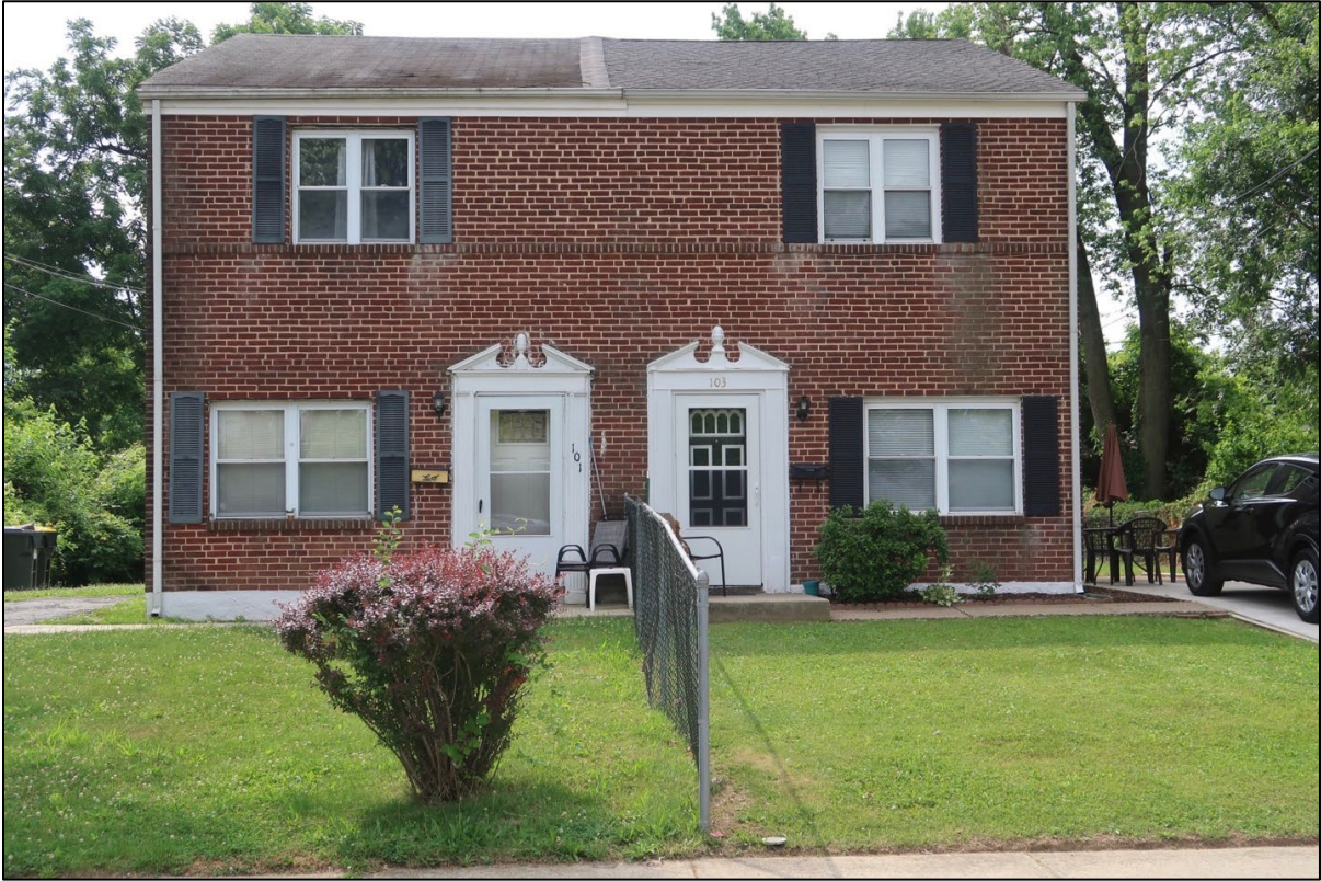
Figure 83. View of a semi-detached, two-family house in Rose Hill Gardens. This is one of the best examples of Early American style architecture in the neighborhood. (Center for Historic Architecture and Design, 2021)
