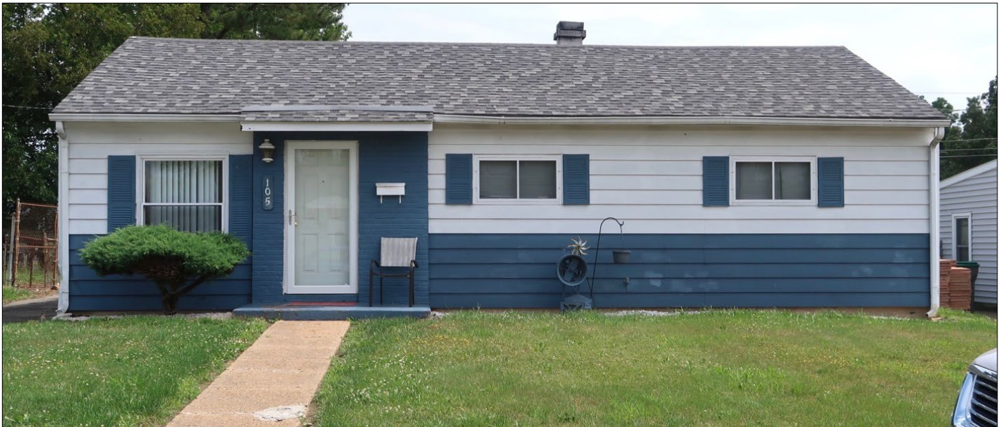
Figure 97. Example of a four-bay, side-gabled ranch house. This was the dominant form constructed in Section 1 of Garfield Park. (Center for Historic Architecture and Design, 2021)
