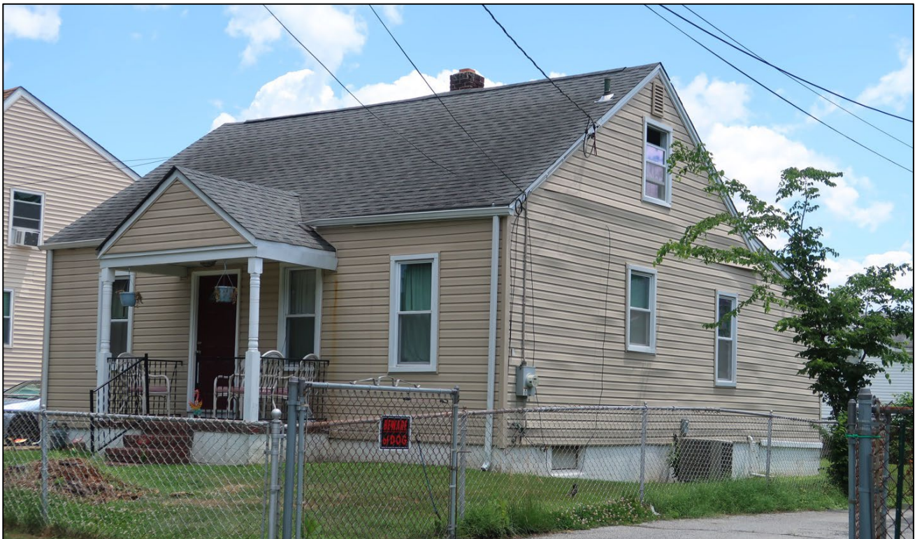
Figure 67. Above is an example of a dormer-less variety of the Cape Cod house form in Mayview Manor. Note the second story window visible on the gable end. (Center for Historic Architecture and Design, 2021)
