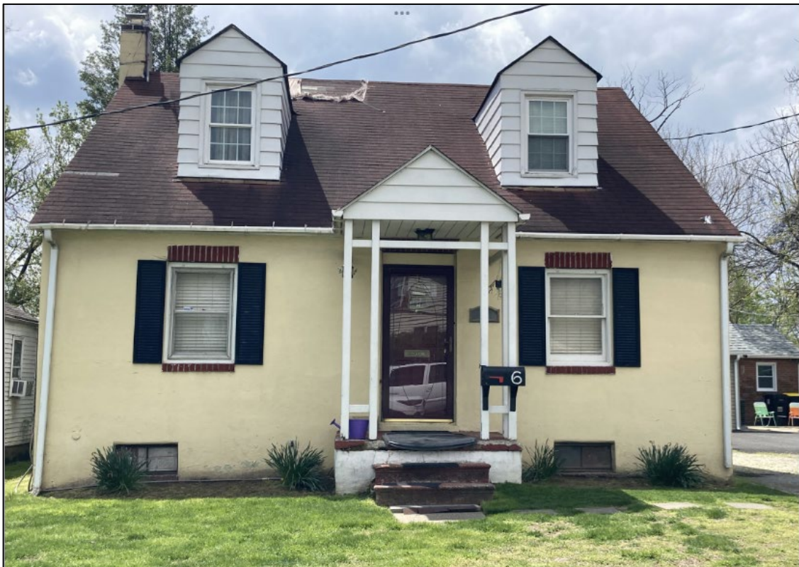
Figure 19. Cape Cod form house in Eden Park Gardens (Center for Historic Architecture and Design, 2022)
