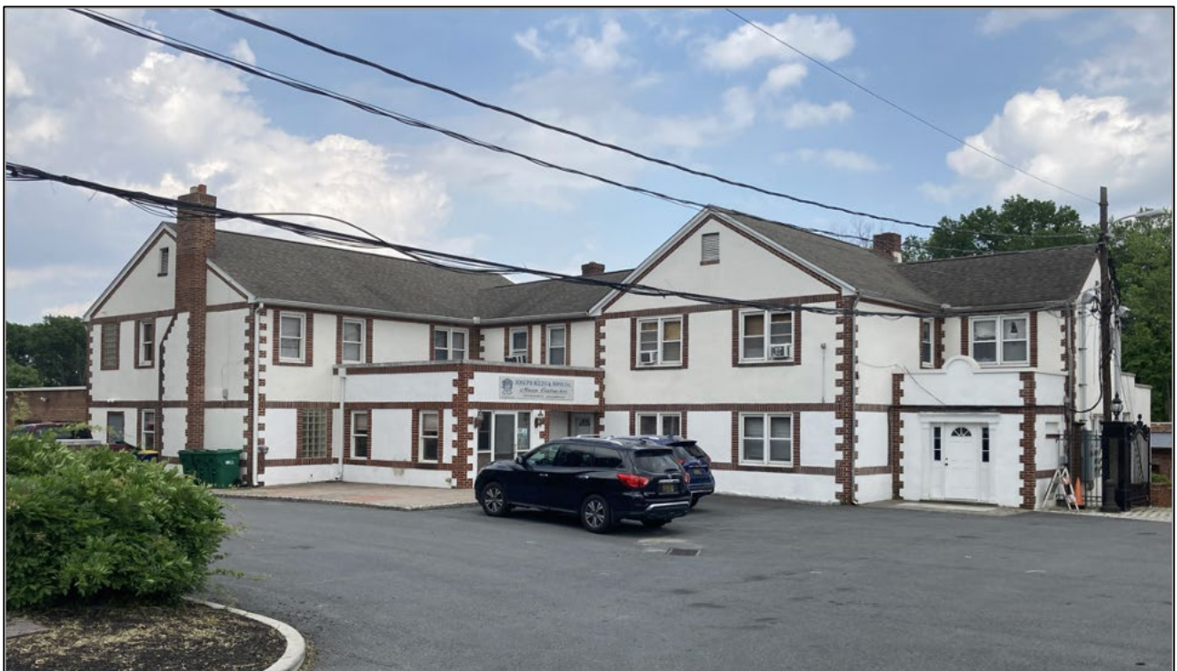
Figure 49. Part of Rizzo & Sons Construction Company complex, Rizzo Avenue. (Center for Historic Architecture and Design, 2022)
