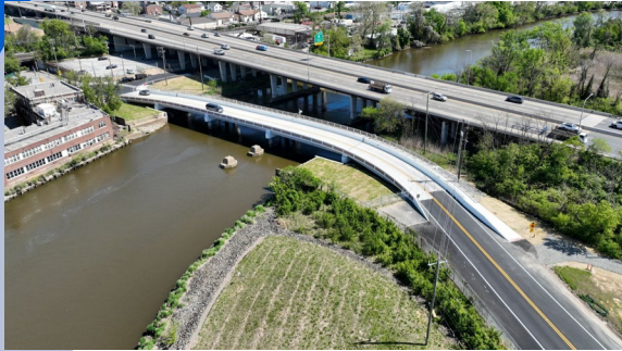
James St. Bridge
