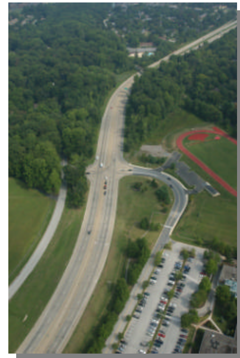
SR141 and Barley Mill Road Intersection
