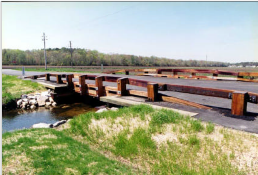
Example of a Timber Bridge
