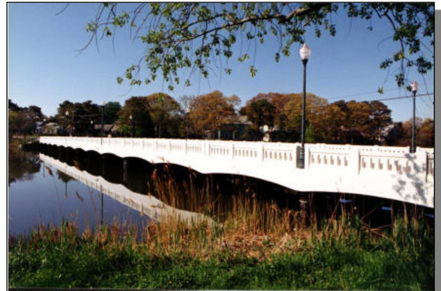
Bridge Over Silver Lake in Rehoboth
