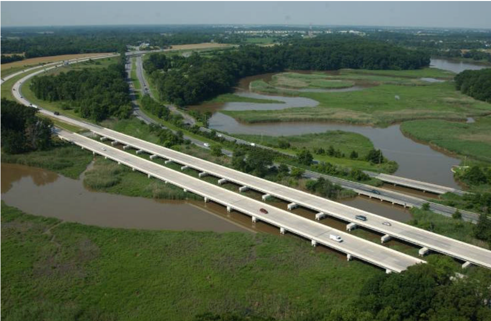
SR 1 Bridges Over Drawyer Creek North of Odessa
