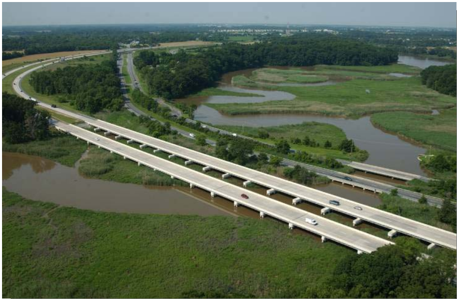
SR 1 Bridges Over Drawyer's Creek North of Odessa
