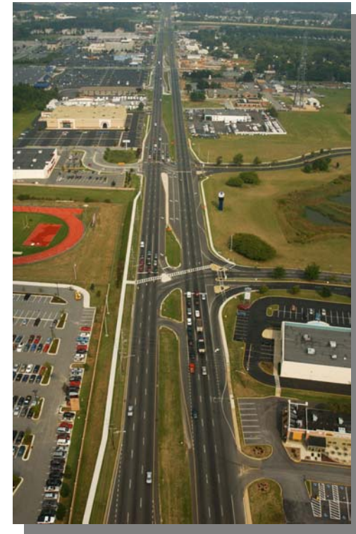
US 13 at Delaware State University Looking North Towards Denney's Road
