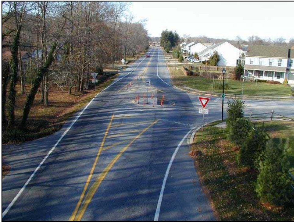
Previous Temporary Traffic Roundabout at Mifflin Road, Dover
