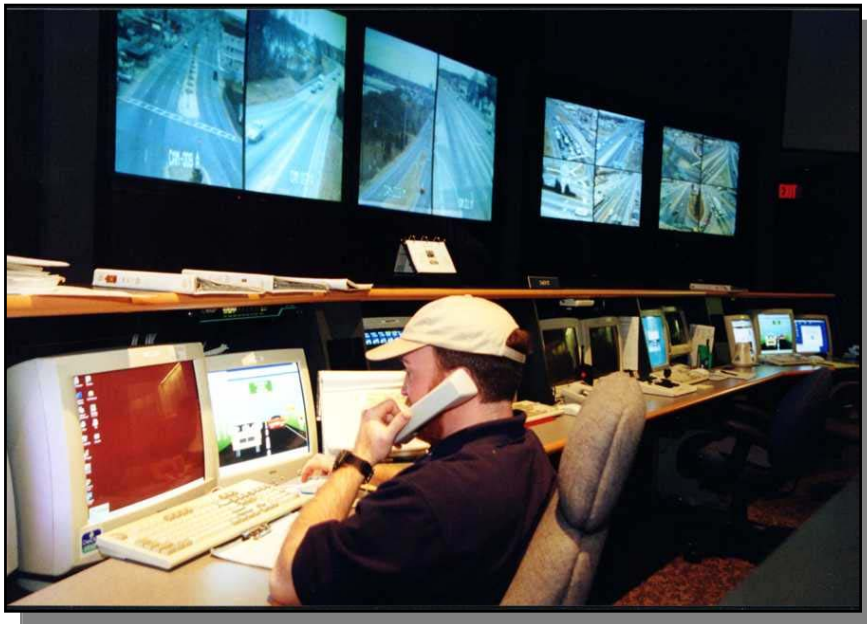
Transportation Management Center in Smyrna
