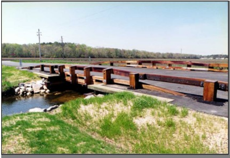
Bridge Over Silver Lake in Rehoboth
