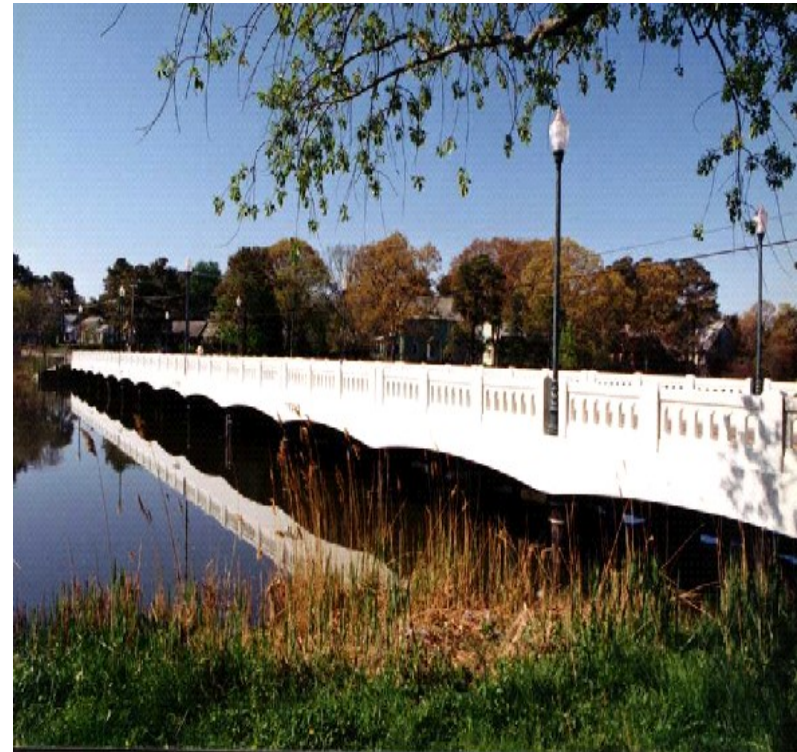
Example of a Timber Bridge
