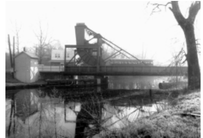
The Central Avenue bridge in Laurel is a patented Scherzer rolling lift bascule bridge, constructed in 1923.
