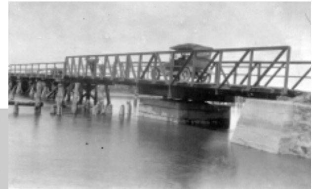
Fennimore's New Bridge (above) and Fennimore's Old Bridge (left), swing span bridges with metal truss superstructures, once carried Thomas Corner Road (State Route 9) over the Appoquinimink River's north and south channels at Fennimores, east of Odessa.
