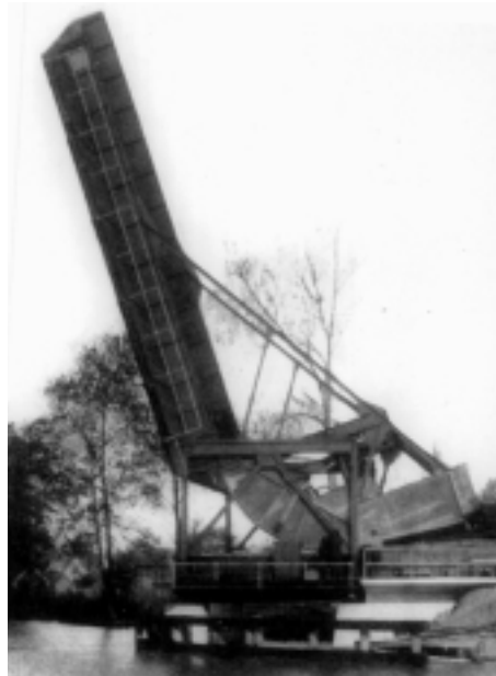
The Central Avenue bridge in Laurel is a patented Scherzer rolling lift bascule bridge, constructed in 1923.
