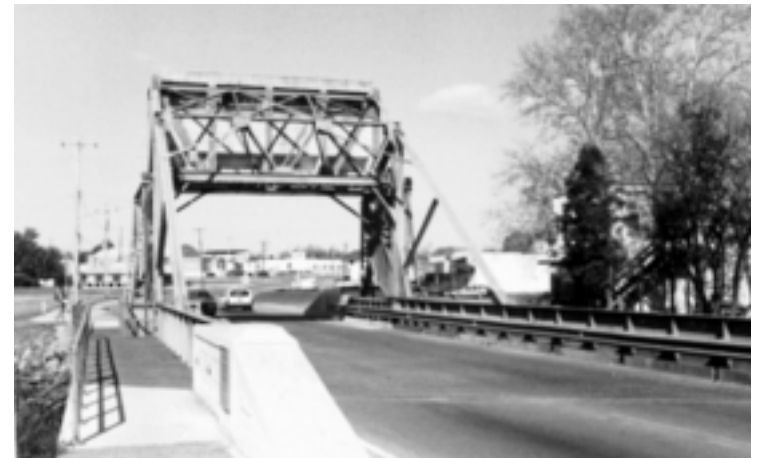
In 1992, DelDOT rehabilitated the Central Avenue bridge. The floorbeams, stringers, and deck were replaced and the concrete abutments and wingwalls repaired. The electrical controls and operators house on the north embankment have been removed, and the bascule span currently is non-operational.
