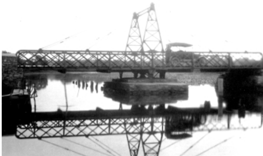
The Blackbird Landing bridge over Blackbird Creek (left) was a variation of swing span bridge with a center tower and cable stays to support the span's free ends in the open position. Similar bridges once spanned over Cedar Creek at Slaughter Beach and the Christina River at Newport. None have survived.
