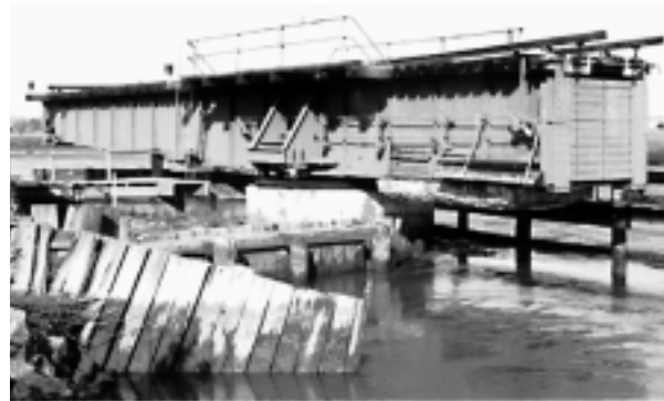
The Lewes bridge, built in 1916, is an example of a bobtail, swing span bridge. This photograph was taken prior to 1996 rehabilitation by DelDOT.
