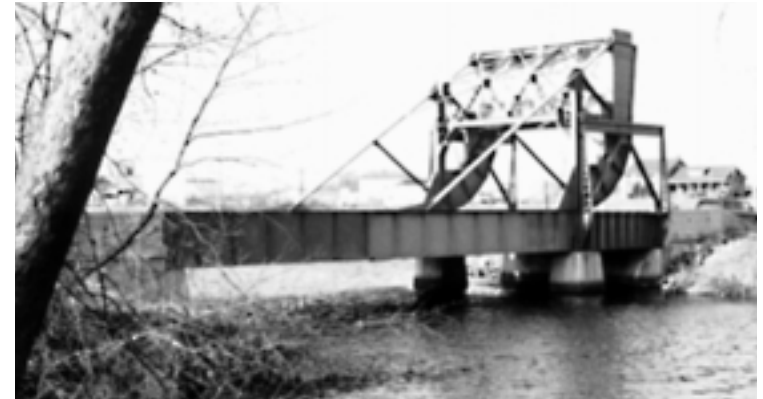
The Central Avenue bridge in Laurel is a patented Scherzer rolling lift bascule bridge, constructed in 1923.
