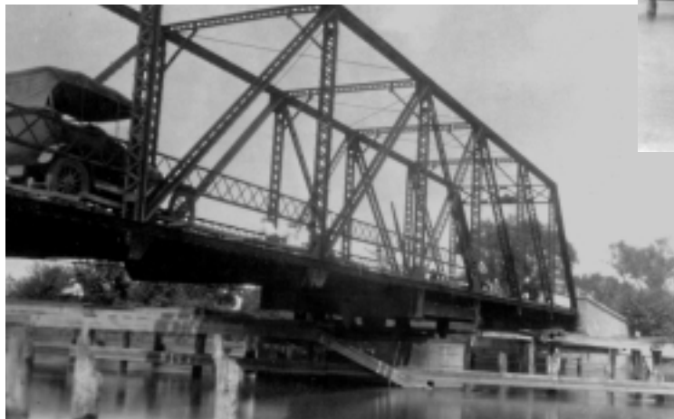
Fennimore's New Bridge (above) and Fennimore's Old Bridge (left), swing span bridges with metal truss superstructures, once carried Thomas Corner Road (State Route 9) over the Appoquinimink River's north and south channels at Fennimores, east of Odessa.
