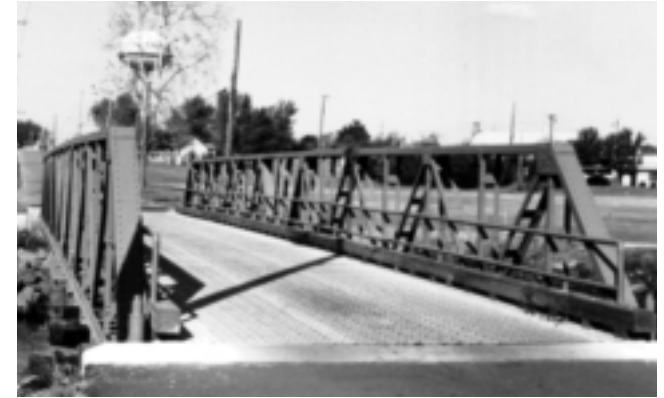
The Poplar Street Bridge (above) is Delaware's only remaining pre-1956 swing span highway bridge.
