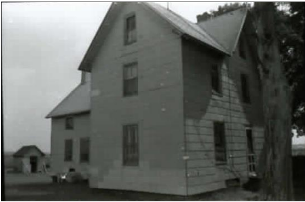
Figure 44: Survey Photo of the House (CRS# S03147) within Area 6.
