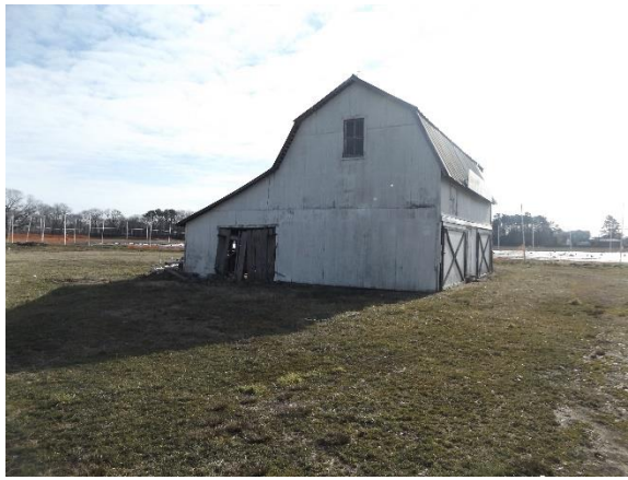
S00975 004 – View of the north elevation of the barn
