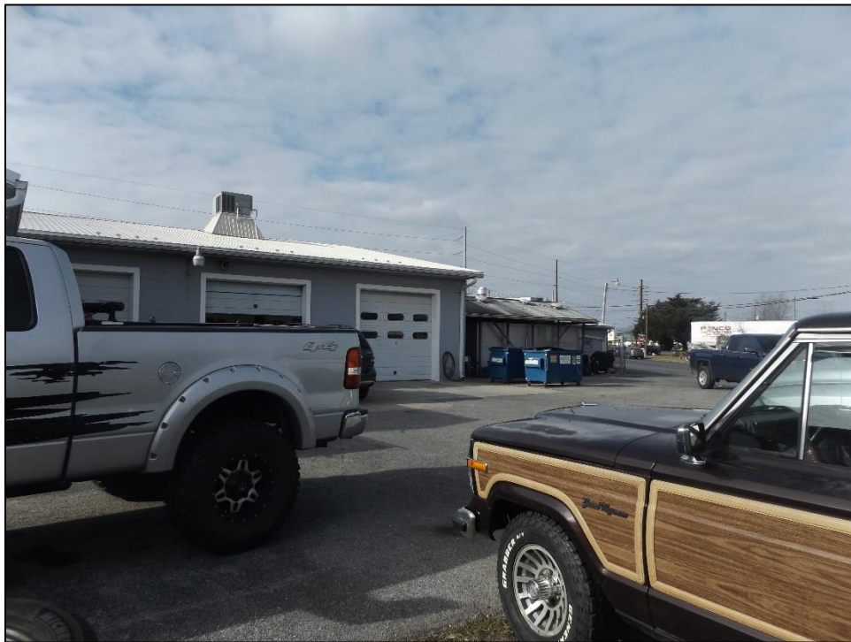
Photo 34: A view of the east elevation (rear) of the building.
