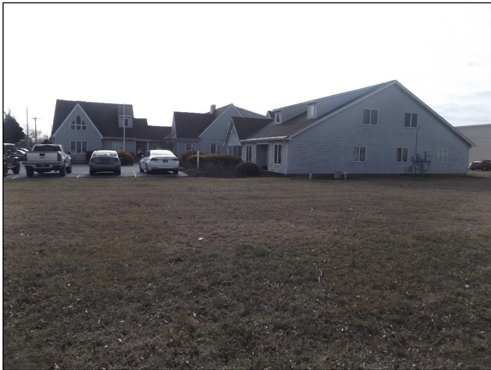
Photo 2: A view of the property looking southeast.
