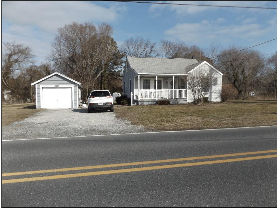
Photo 25: A view of the primary (south) façades of the main house and garage.
