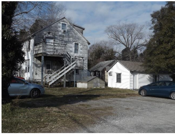
S00979 004 – View of east elevation of the main house. A rear shed-roofed addition can be seen on the north elevation. The south elevation on House A can be seen in the right section of this image. In the center, the south and east elevations of House B can be seen in the background.
