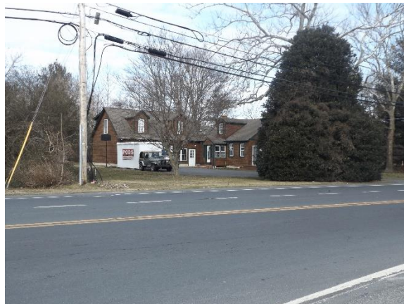
S13307 003 – Detail view of the recessed section of the house and the south elevations
