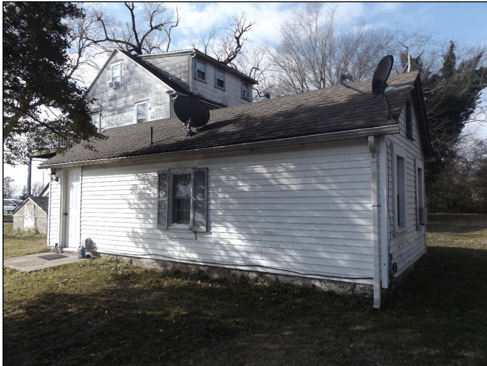
Photo 18: A view of the primary (east) façade of "House A." The shed-roofed dormer on the rear (north) elevation of the main house can be seen here.
