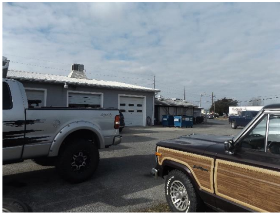
S13306 005 – View of the rear (east) elevation of the property, including the rear of the Fully Belly Bistro section of the building
