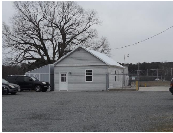
S00976 004 – A view of the storage building on the southeast corner of the property
