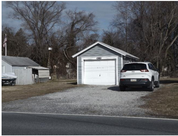
S13327 004 – Detail view of the primary (south) façade of the detached garage
