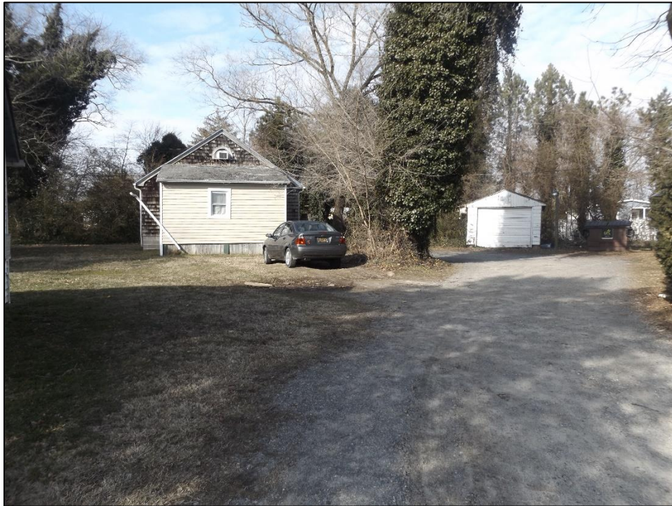
Photo 20: A view of the east elevation of "House B," where the shed-roofed lean-to addition can be seen. The small garage on the property can also be seen to the right.
