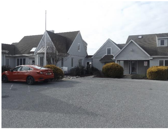
S00973 004 – Detail view of the northeastern elevations of the structures, where the multiple office entrances and connecting breezeway can be seen.
