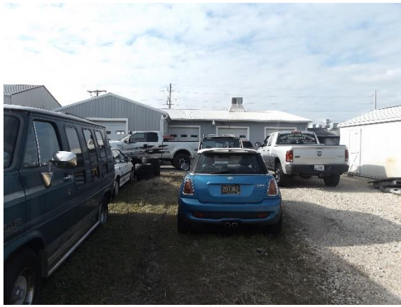
S13306 004 – View of the rear (east) elevation of the C.J.'s Beach Bays Service Center section of the property
