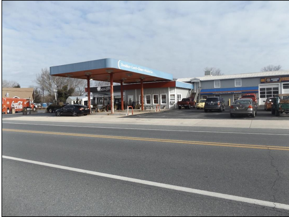
Photo 31: A view of the primary façade of the property looking north from Wescoats Road.
