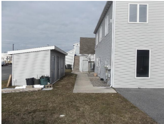
S00973 009 – A view of the three doors on the façade of the shed structure located behind the main house.
