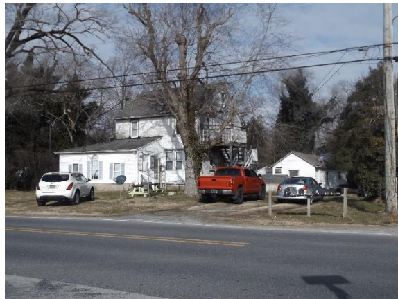
S00979 003 – View of primary (south) and east elevations of the main house
