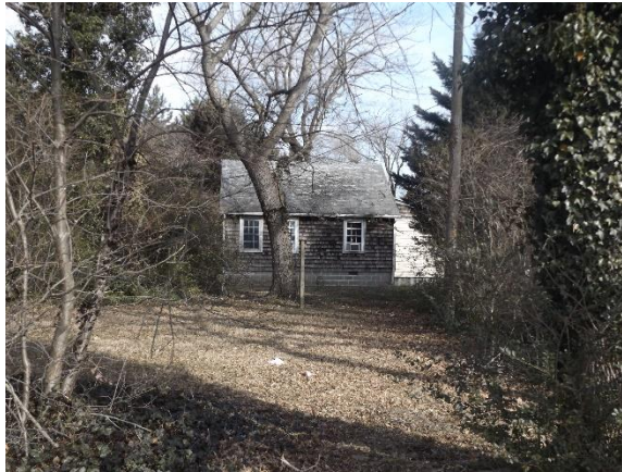
S00979 006 – View of south elevation of House B, as it was referred to in 1979 photographic documentation.
