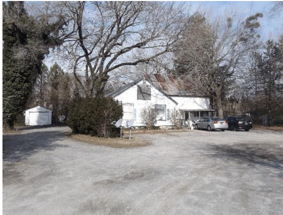
S00979 008 – View of primary (south) façade of House C, as it was referred to in 1979 photographic documentation. The small garage on the property can also be seen to the left.
