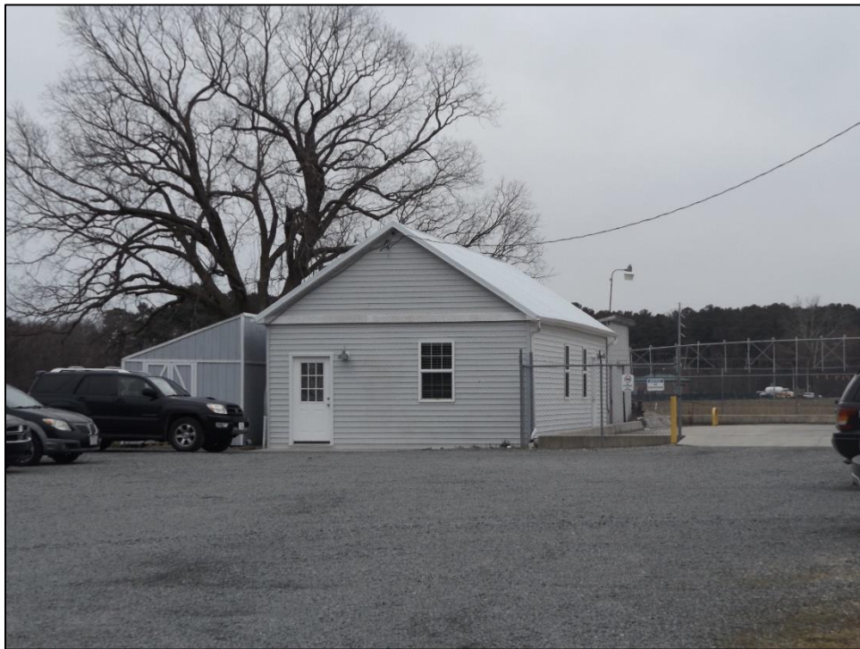
Photo 13: A view of the storage building located on the southeast corner of the property.
