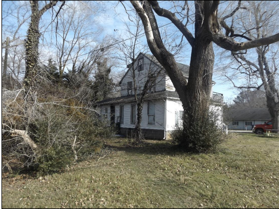
Photo 15: A view of the west elevation of the main house, which shows the extent of the one-story addition.
