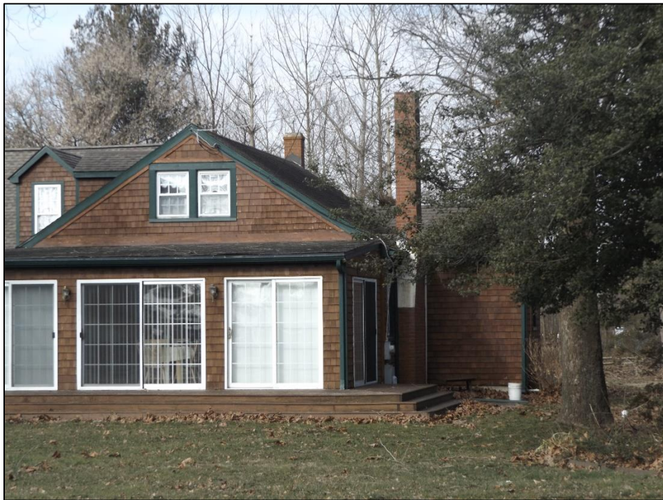
Photo 37: A detail view of the primary façade with its enclosed porch and the north elevation.
