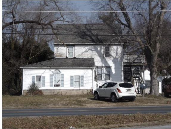
S00979 001 – View of primary (south) façade of the main house on the property
