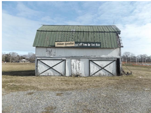
S00975 003 – View of the primary (west) façade of the remaining barn on the property
