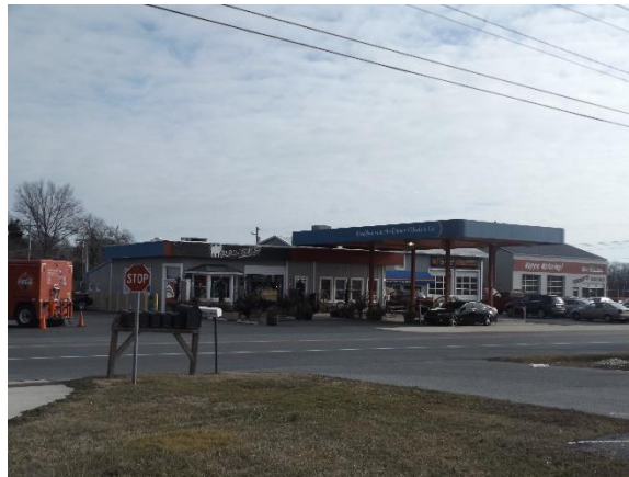
S13306 002 – View of the property looking east from Wescoats Road
