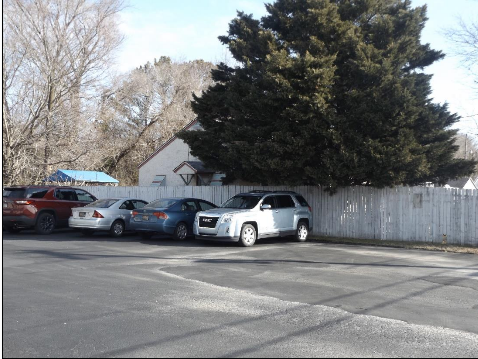
Photo 30: A view of the west elevation of the house. Much of this is obscured by vegetation and the wooden fence.
