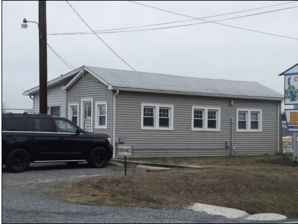
Photo 12: A view of the north and east (primary) elevations showing the entrance to the office.
