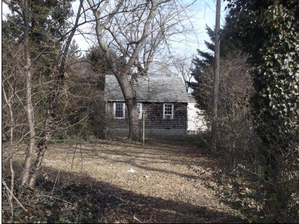
Photo 19: A view of the south elevation of "House B."
