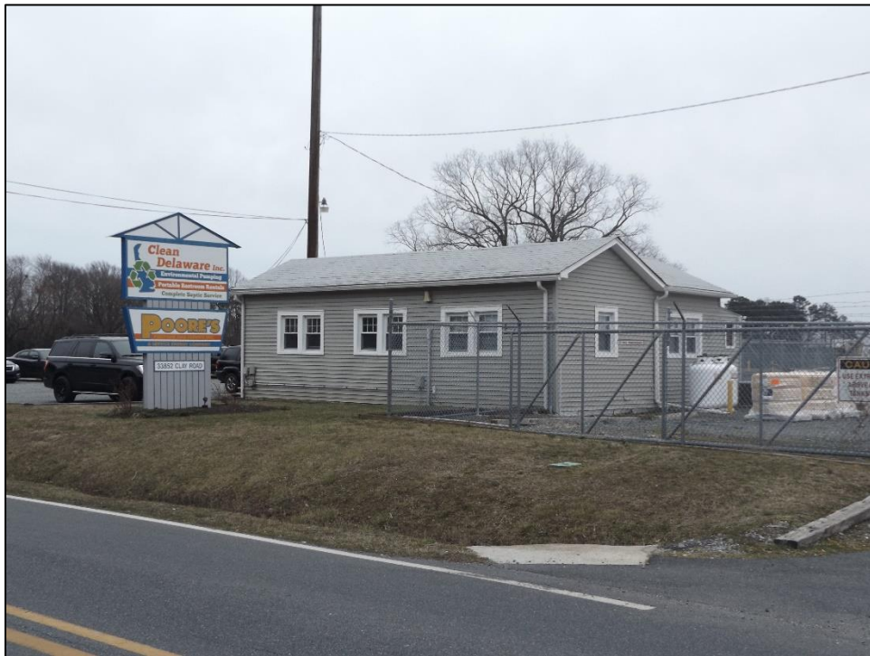
Photo 11: A detail view of the west and north elevations of the main office building.
