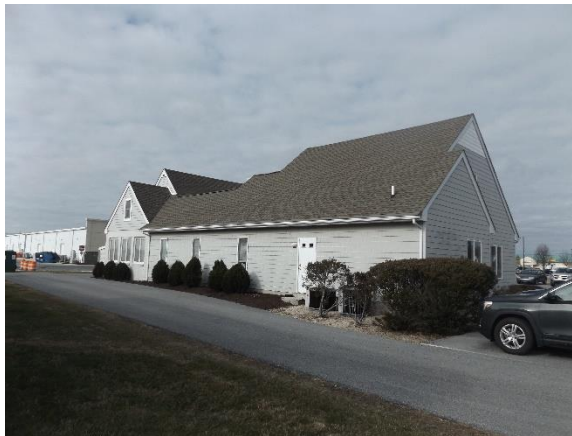
S00973 006 – View of the southern elevation and driveway on the large addition to the original house.
