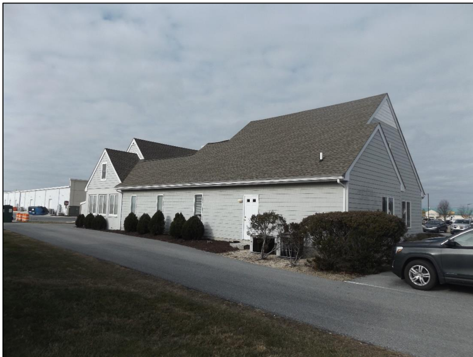
Photo 6: A view of the southern elevation and driveway on the large addition to the original house.
