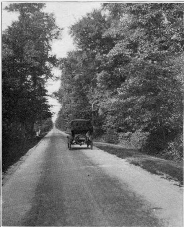
DUPONT BOULEVARD NEAR MILFORD Before marking center line. Observe lack of separation of oil dripping into distinct lanes as shown below.
