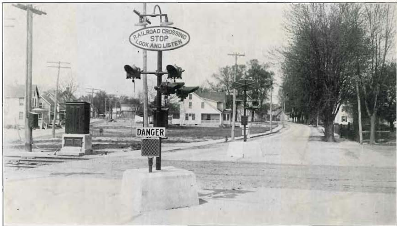
EXCELLENT GRADE CROSSING PROTECTION BY FLASHING SIGNALS INSTALLED BY PENNSYLVANIA RAILROAD AT MILLSBORO
