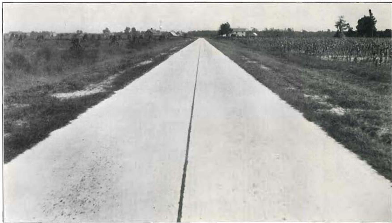
LAUREL-SHARPTOWN ROAD, SUSSEX COUNTY SHOWING NON-METALLIC CENTER-JOINT. NOTE EXCELLENT ALIGNMENT OF JOINT
