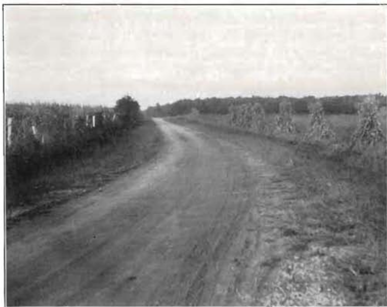
WHITE OAK ROAD, KENT COUNTY SECONDARY ROAD— SLAG-CLAY TYPE
