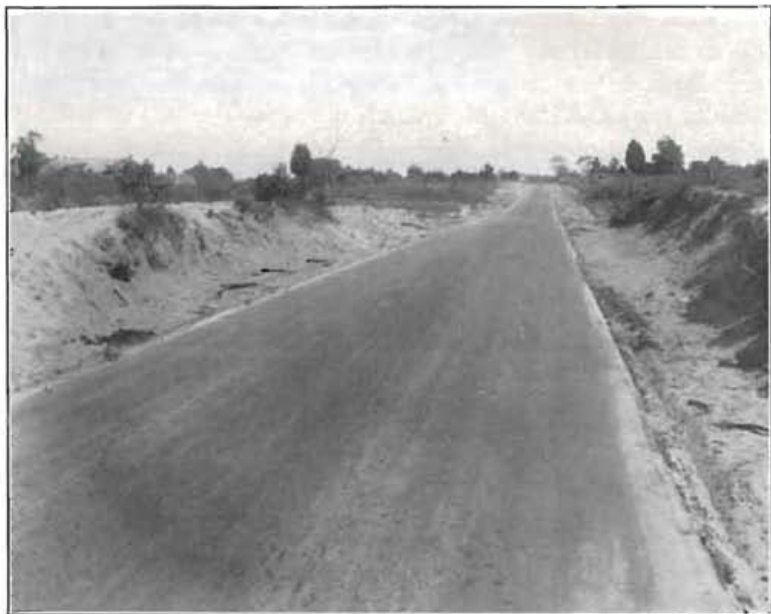
SAND-ASPHALT ROAD NEAR CONCORD, SUSSEX COUNTY. COMPLETED PAVEMENT; SHOULDERS UNFINISHED
