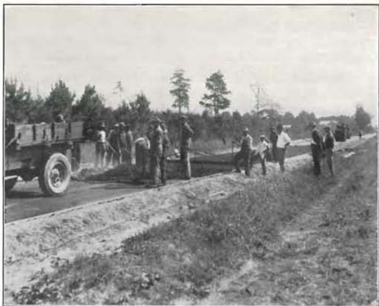
SAND-ASPHALT ROAD, SUSSEX COUNTY DURING CONSTRUCTION
