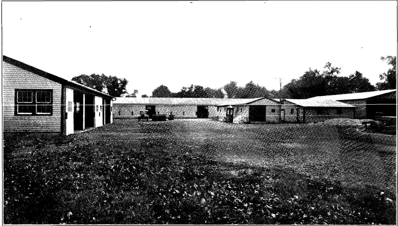
STATE HIGHWAY REPAIR SHOP AND GARAGE AT DOVER. AUTOMOBILES, TRUCKS, MOTORCYCLES AND MAINTEN- ANCE EQUIPMENT ARE REPAIRED AND STORED HERE.
