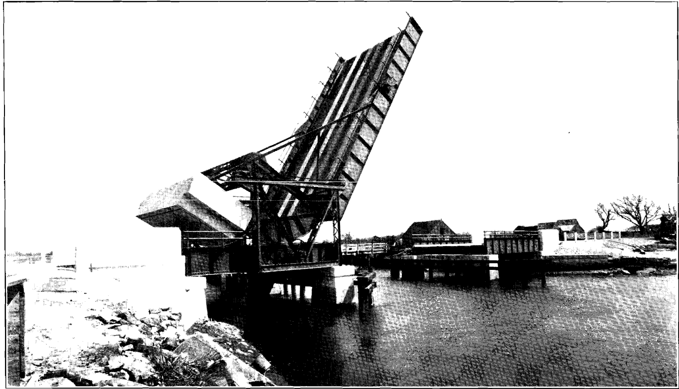
BROADKILL BRIDGE. DRAW SPAN OPEN. THE OVERHEAD COUNTERWEIGHT TYPE CAN BE BUILT AT LESS COST THAN THE PIT COUNTERWEIGHT TYPE WHERE APPEARANCE IS OF SECONDARY CONSIDERATION.
