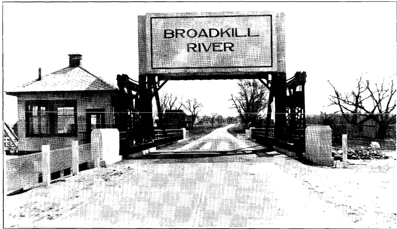
BROADKILL RIVER BRIDGE, SUSSEX COUNTY, ROLLING BASCULE BRIDGE WITH OVERHEAD COUNTERWEIGHT. COMPLETED, 1927.
