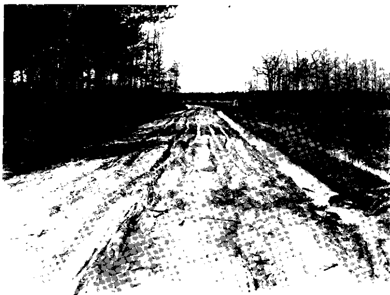
Farmington-Fisher's School Road, Kent County. Before Construction.
