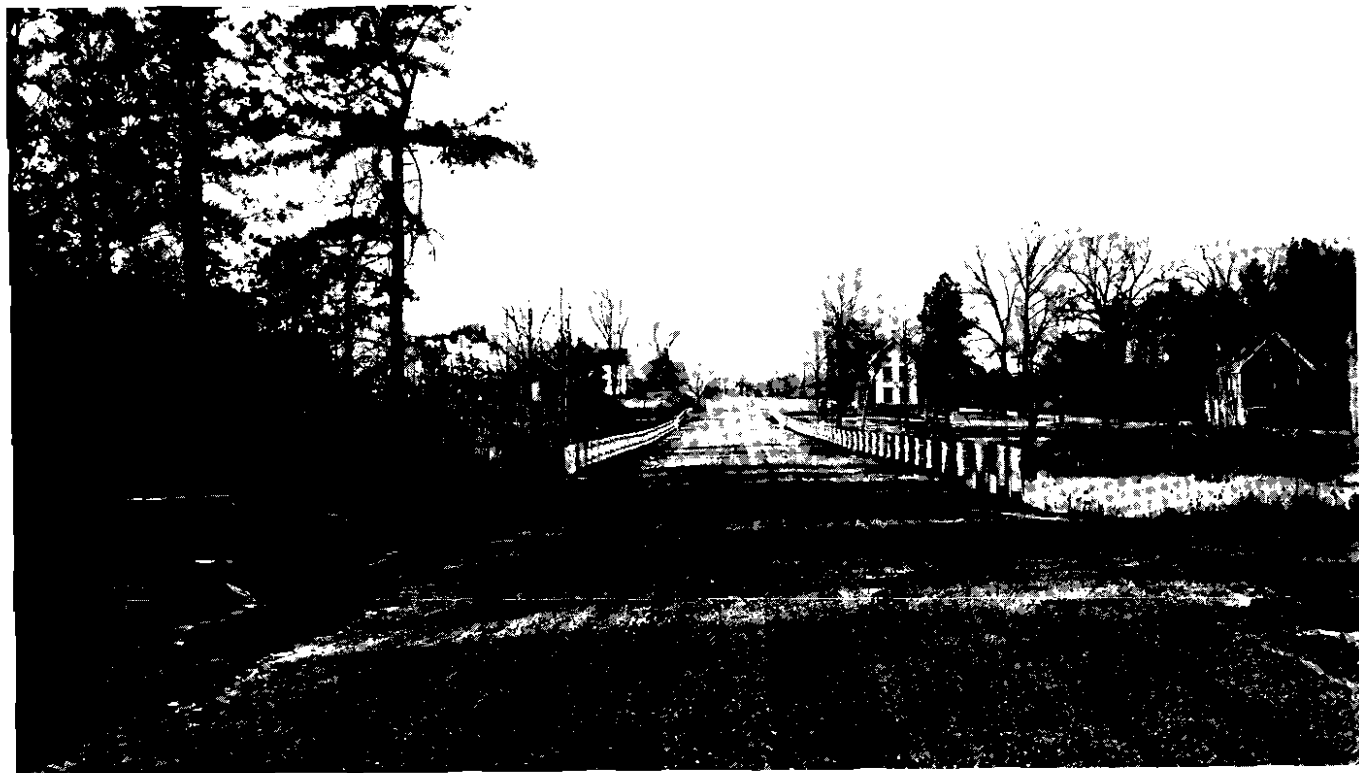
Lincoln City-Waples Pond State Highway, Sussex County. Secondary traffic bound slag road.
