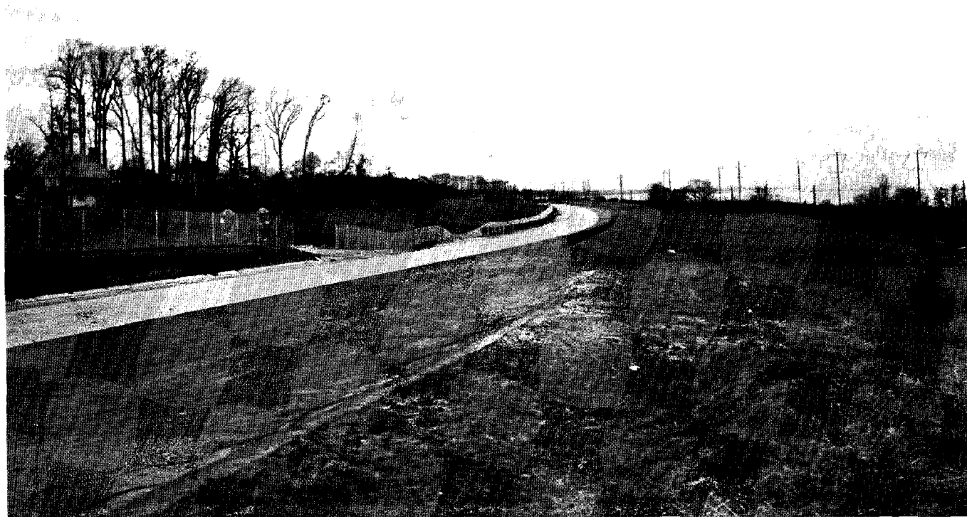
New Castle County—"Northeast Boulevard" near Wilmington
