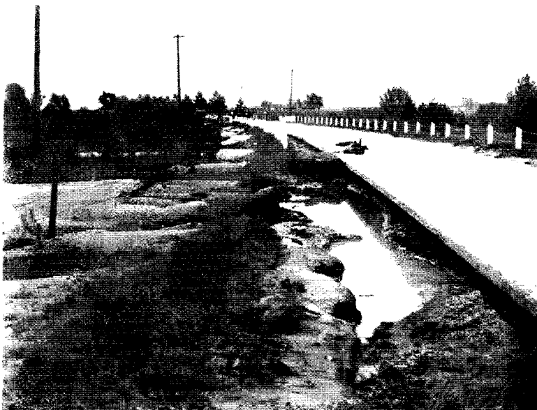
Kent County—Typical washout during September storm
