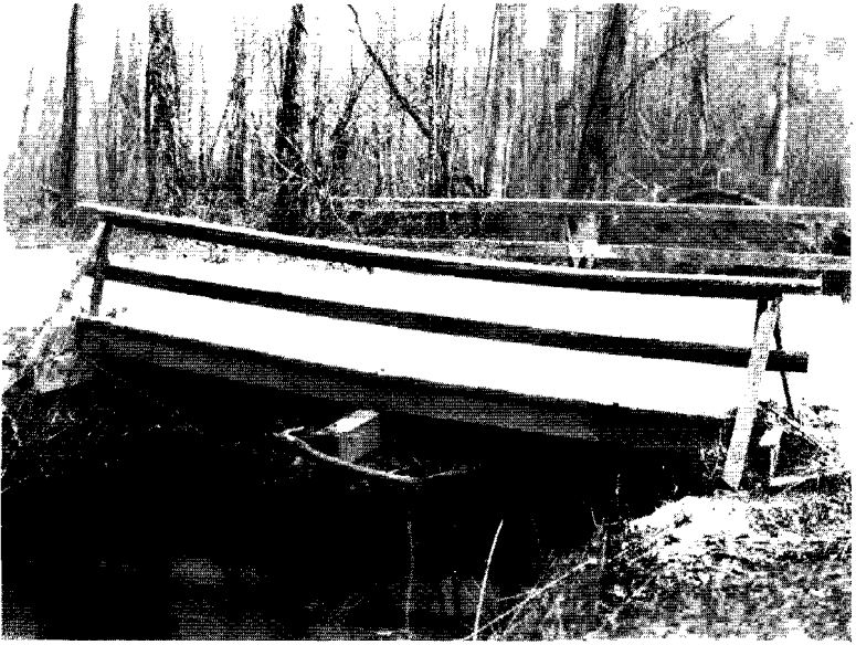
Approximately a hundred county bridges of this type were washed out by the storm of September, 1935 and —
