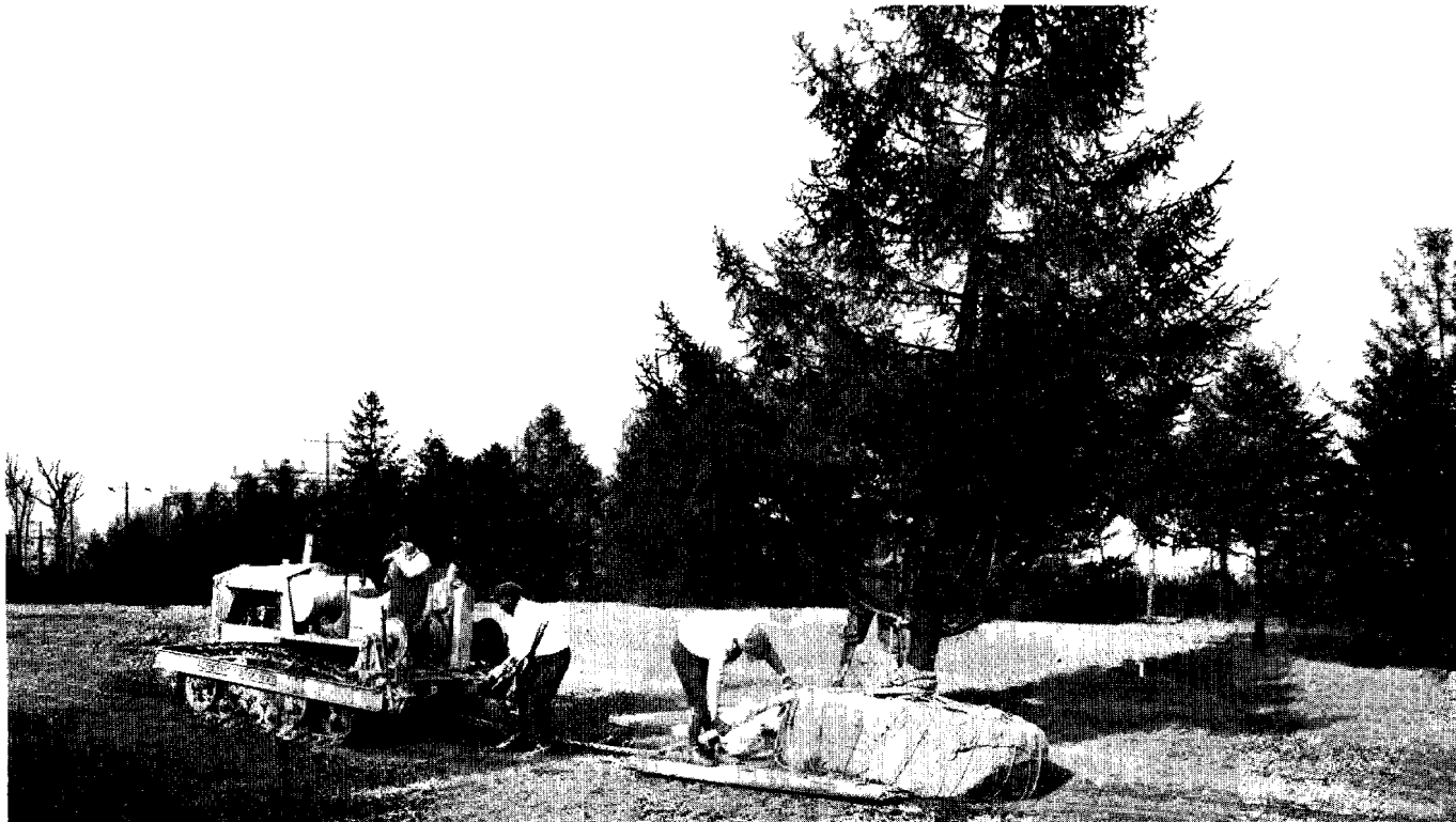
"Northeast Boulevard" north of Wilmington. Removing lawn trees from Right of Way. New Castle County
