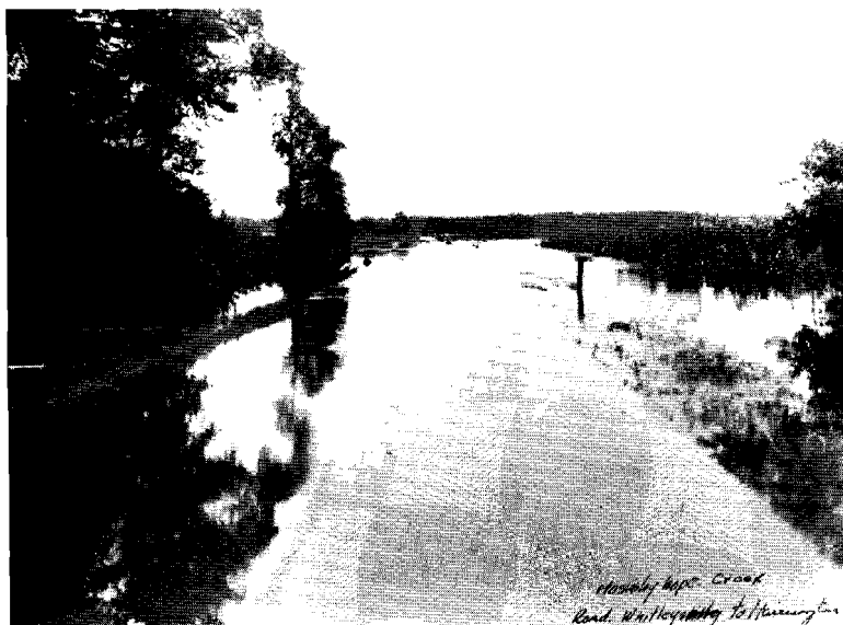
Marshy Hope Creek Bridge. Harrington to Whiteleysburg, September, 1935
