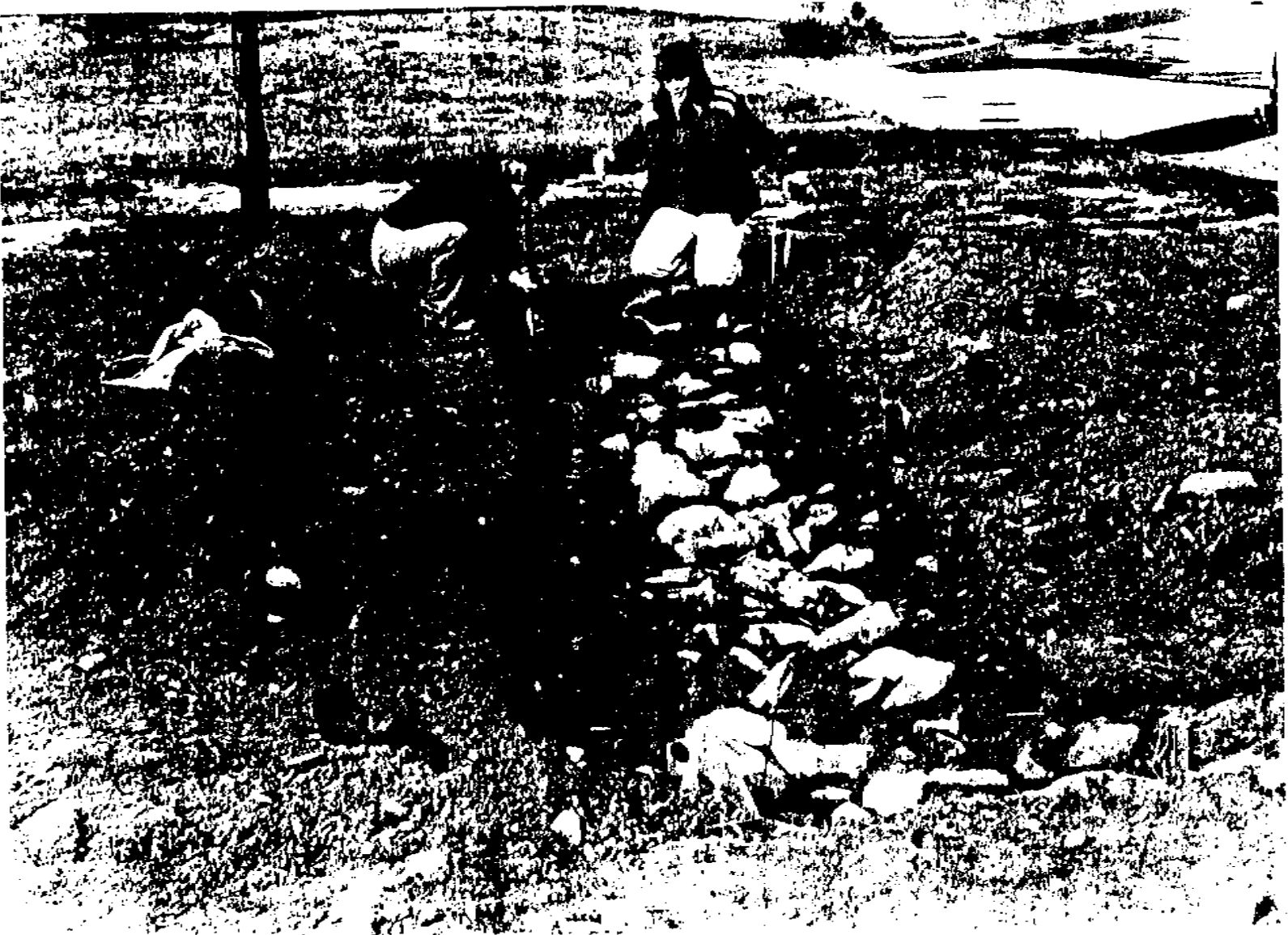
Plate 3: Upper Foundation, During Testing
