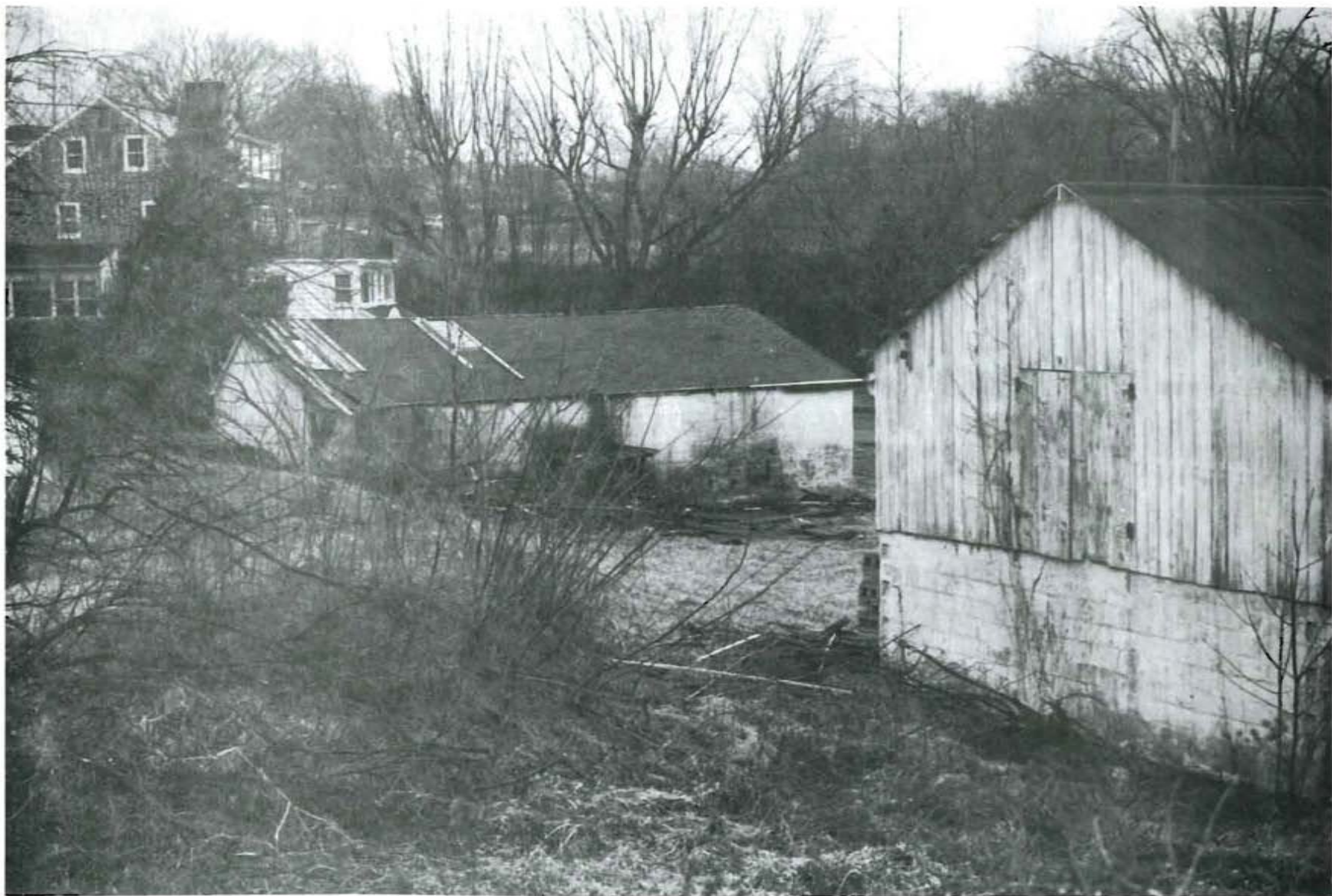
PLATE 23: Garage and Stable at Chandler House, View to Southeast
