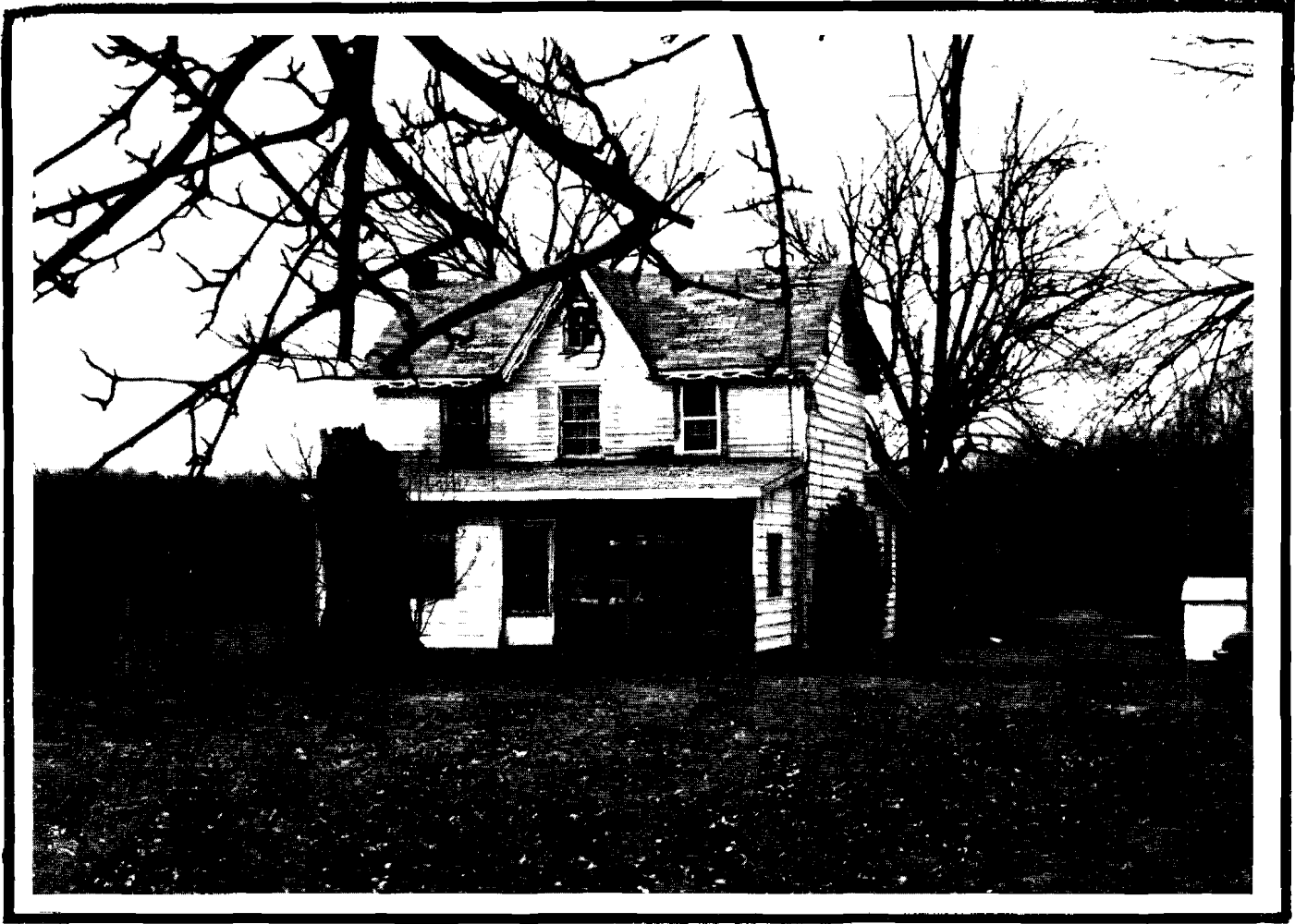
PLATE 3: Jonathan Davis House, View to West
