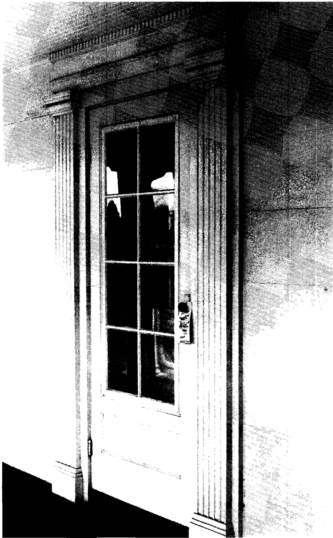
PLATE 8: Silver Hill Farm, Farmhouse, Main Entrance
